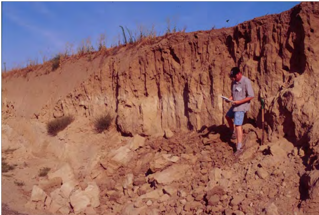
Figure 9. Photograph of a Typical Loess Embankment Exposed in a Road Cut
