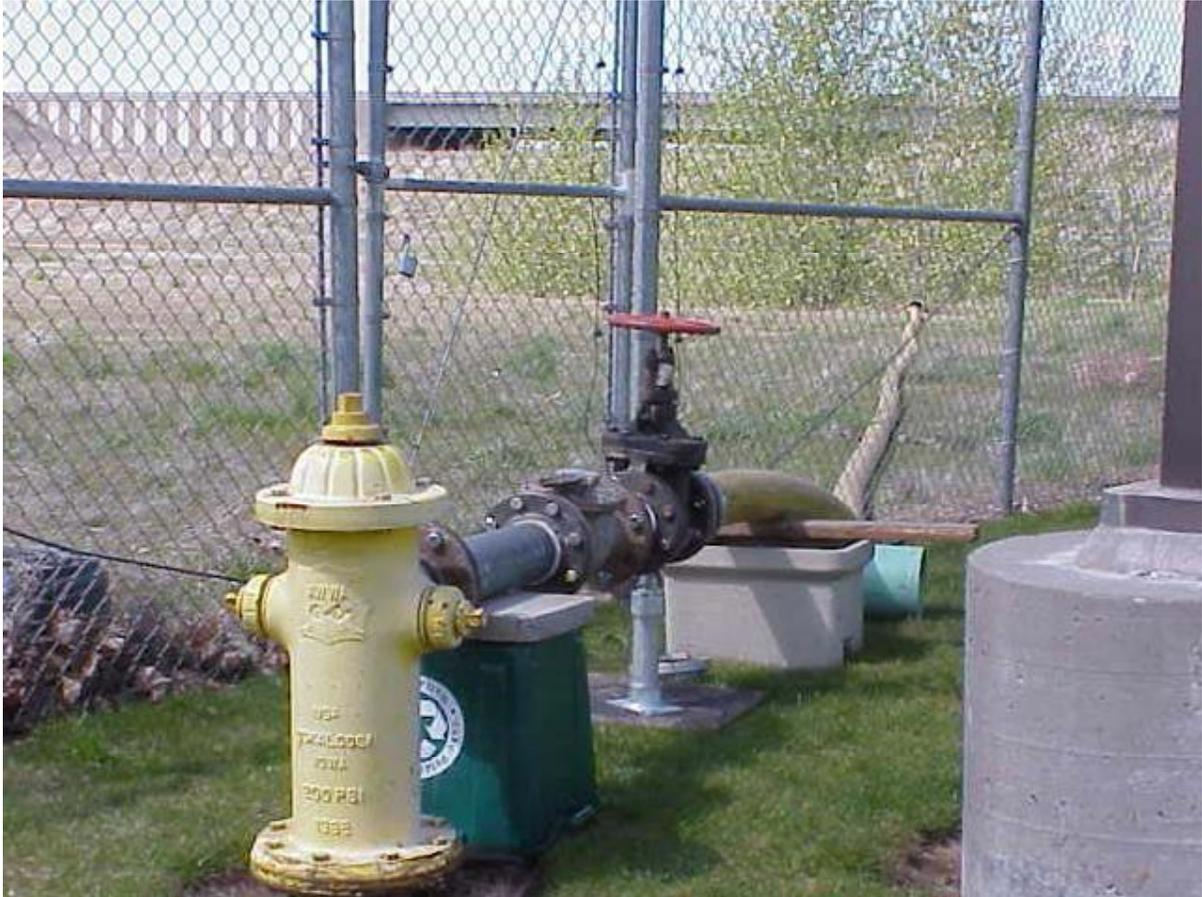
**FIGURE 5-1. Test Setup at Hydrant**
