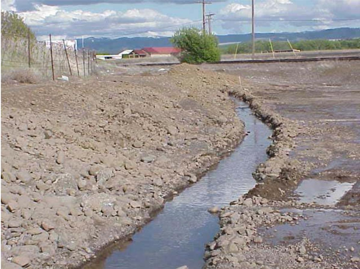
**FIGURE 5-17. Seepage from Cut Bank**
