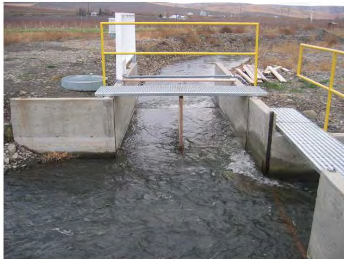
Figure 10. HBDIC Recharge Project Intake Structure in Operation (Spring, 2005)
