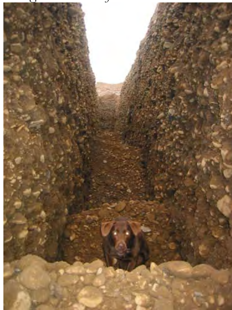
Figure 2. (2/8/5) Photo taken in trench created while constructing spreading basin. "Rust colored rocks clearly evident in trench bottom. (Dog "Kenai" in picture for scale).
