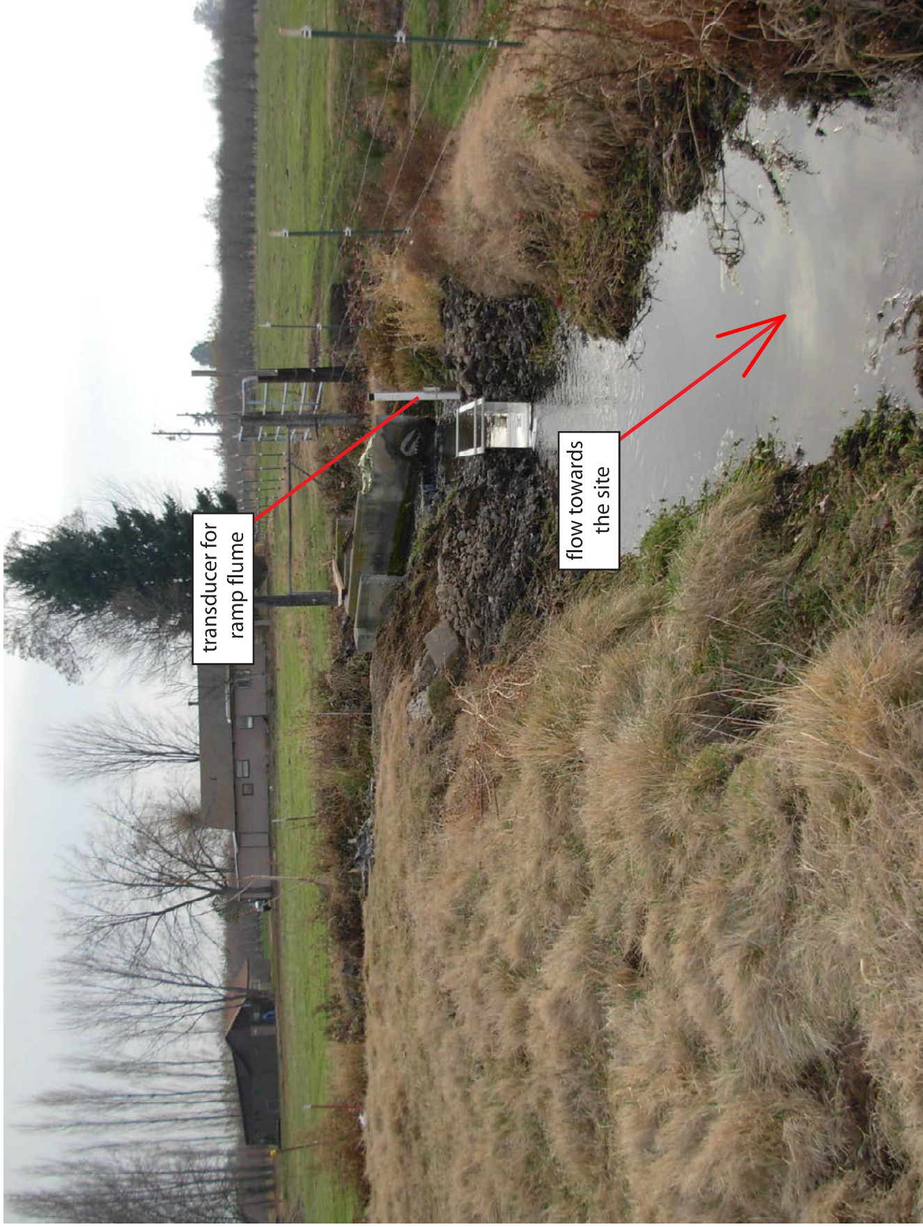
Figure 5. Photograph of branch ditch ramp flume just below the diversion off Wells Ditch.
