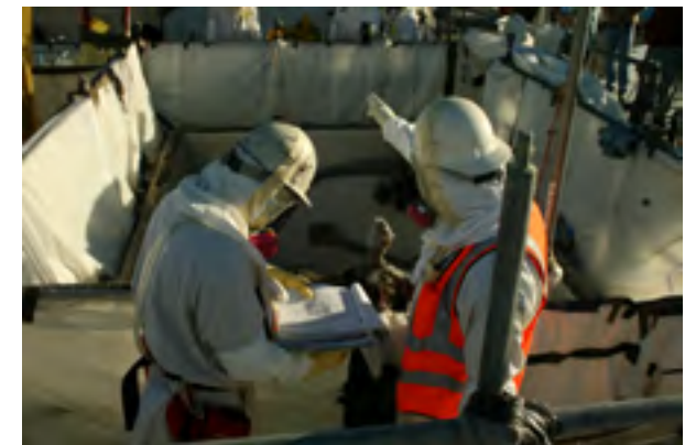
Staff evaluating a workplan for installing a tank farm pump.
