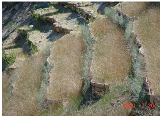
Use of biosolids in slope stabilization along U.S. Highway 97A in Chelan County (background, no biosolids; foreground, biosolids compost)
