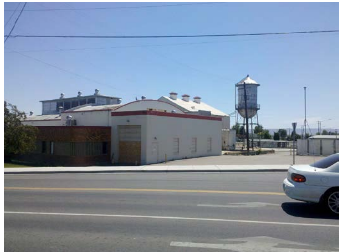
View of the Site from the North
