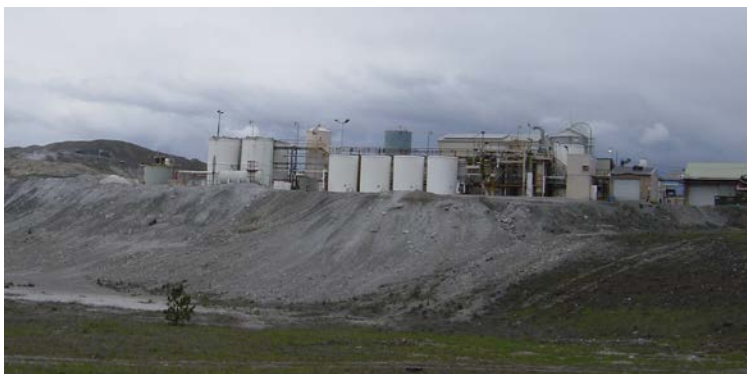
Looking North at the Site from Sullivan Road
