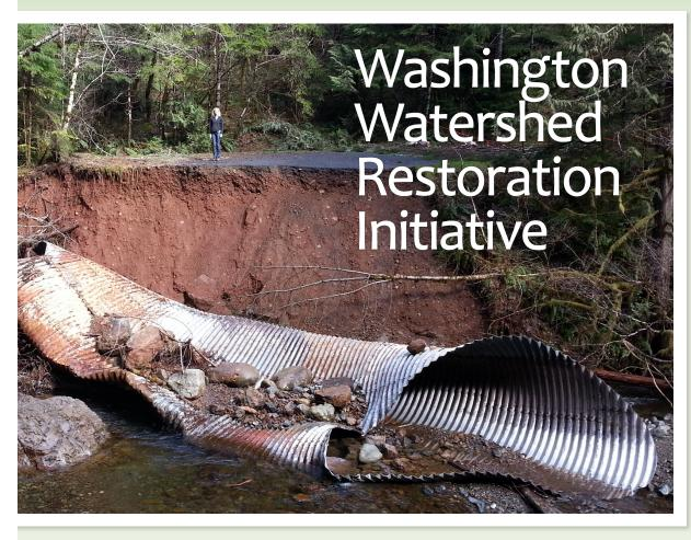
◀ This 13-foot diameter culvert became plugged with forest debris during a rain-onsnow storm event in the Olympic National Forest in the winter of 2012. The stream was forced to flow over the road fill, washing it away and depositing sediment downstream as far as Hood Canal. More high intensity storms lead to more damage to the National Forest road system. Wildlands CPR photo
