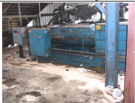
Recycling machinery with evidence of fluid leaks and debris
