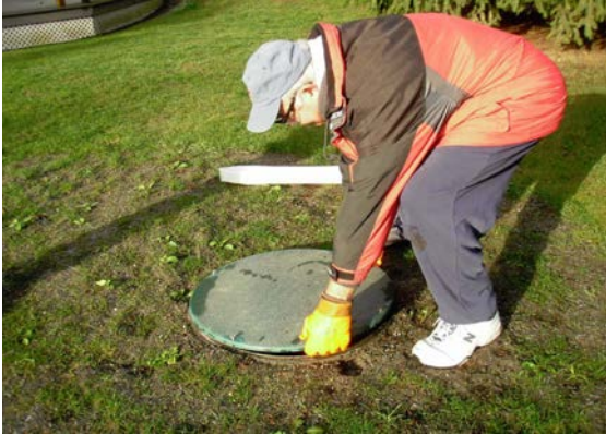
Man inspecting his septic tank
