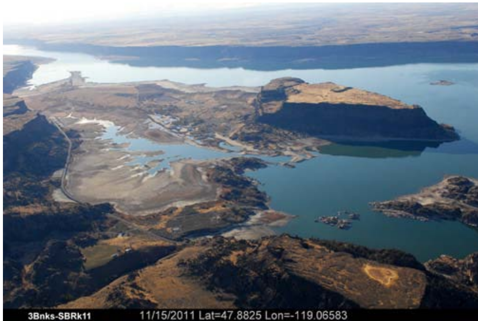
Photograph 4-6. Illustration of a reservoir drawdown, or bathtub ring conditions. This is a photo of Banks Lake reservoir at Steamboat State Park during approximately 33-foot maintenance drawdown (November 11, 2011).
