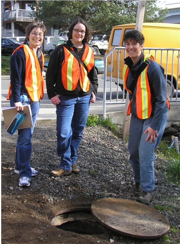
Water Quality Program staff (left to right) Sarah Davenport-Smith, Rachel McCrea, and Anne Dettelbach inspect a stormwater catch basin to ensure it is functioning properly.
