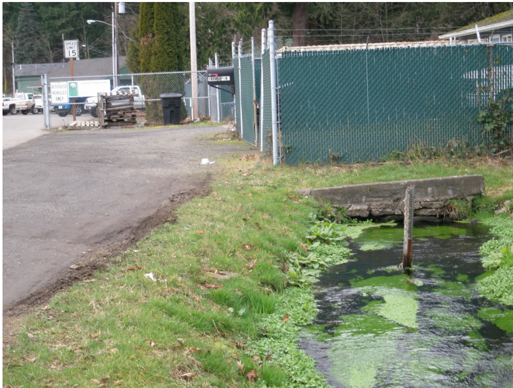
Figure B7. Unnamed Tributary to Shelton Creek, Daylights at the City Animal Shelter.
