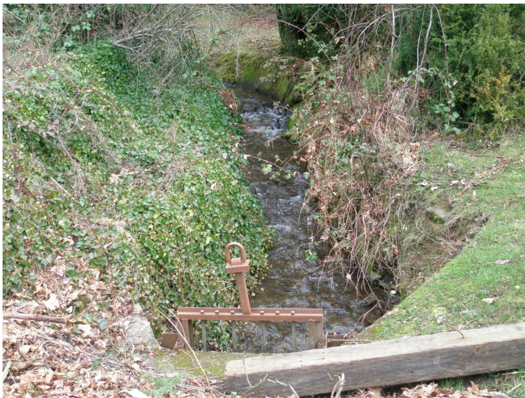
Figure B6. Canyon 3, Upstream of the Northcliff Road.
