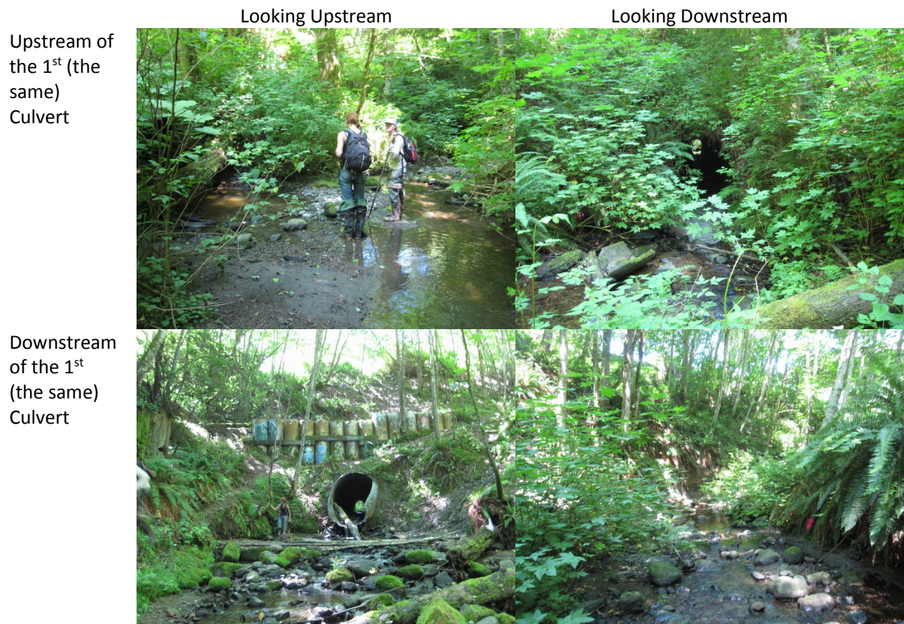
Figure 7. A comparison of immediately upstream and immediately downstream of the first culvert that conveys Peabody Creek under a road on the upstream end of the impaired reach.
