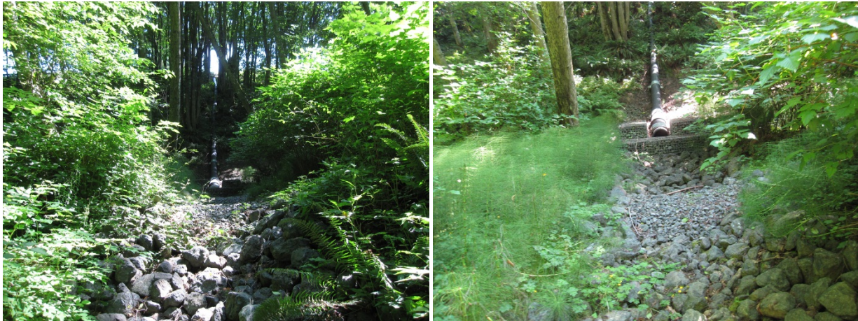
Figure 8. Structures built to convey stormwater from streets adjacent to Peabody Creek.
