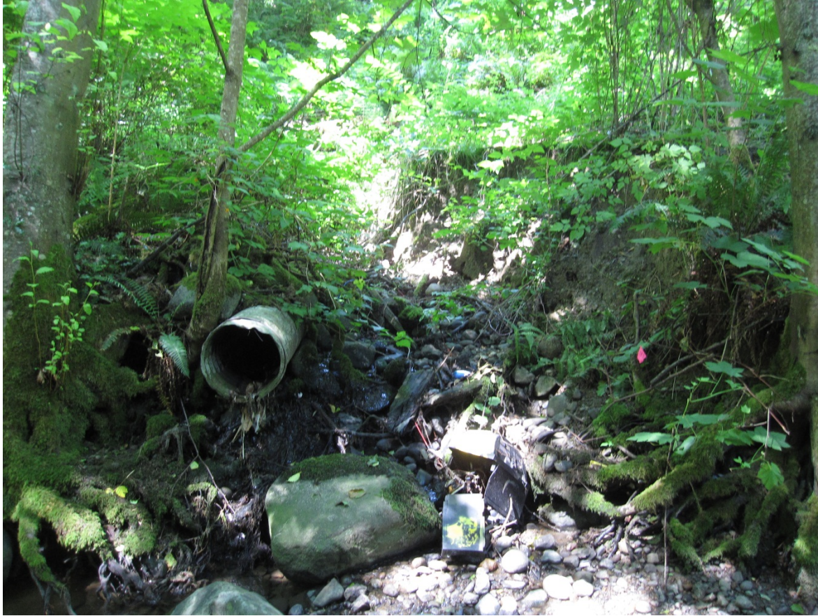
Figure 6. Culverts are not effectively conveying runoff to the stream.
