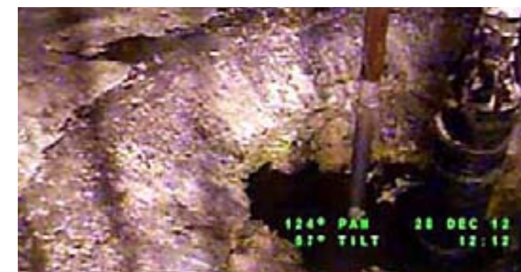
Probe in tank BY-102 measuring the supernatant (liquid waste) level.
