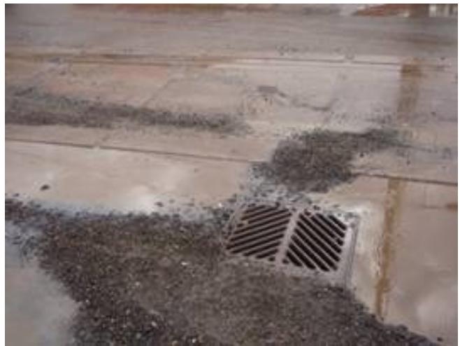
Stormwater runoff entering a storm drain. Runoff can carry soil pollutants like arsenic and lead.
