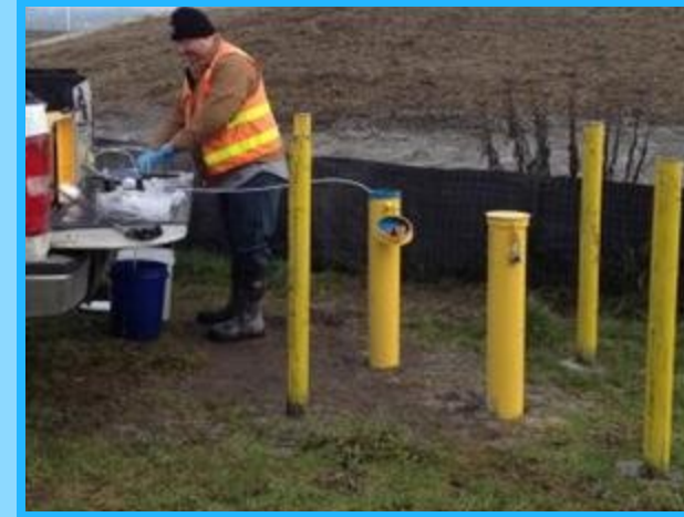
Groundwater sampling at newly installed monitoring wells.
