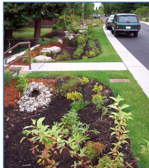
Bioswale photo courtesy of the Washington Stormwater Center
