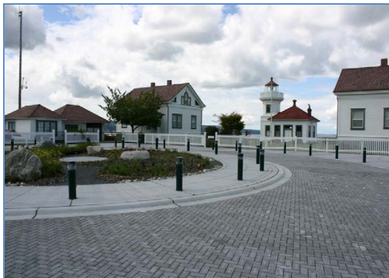
Permeable Pavers photo courtesy of the Washington Stormwater Center
