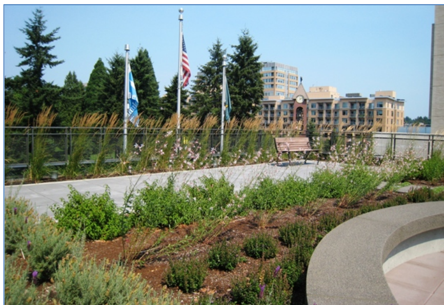
Green roof on top of The Columbian newspaper building in Vancouver, Washington.
