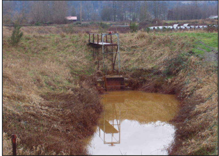
Batt Slough prior to new tidegate installation
