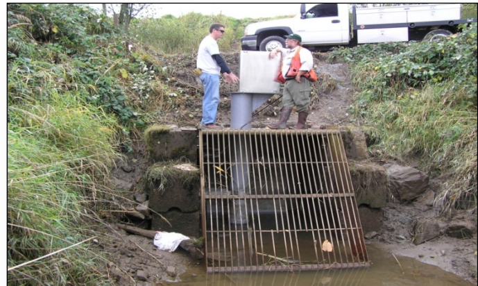
Bob Penhale inspects the final tidegate
