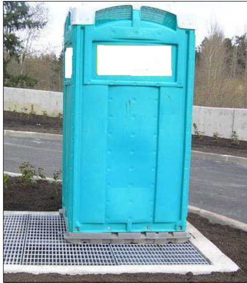
Figure 33. Portable toilets at construction sites need proper maintenance and location away from surface waters.
