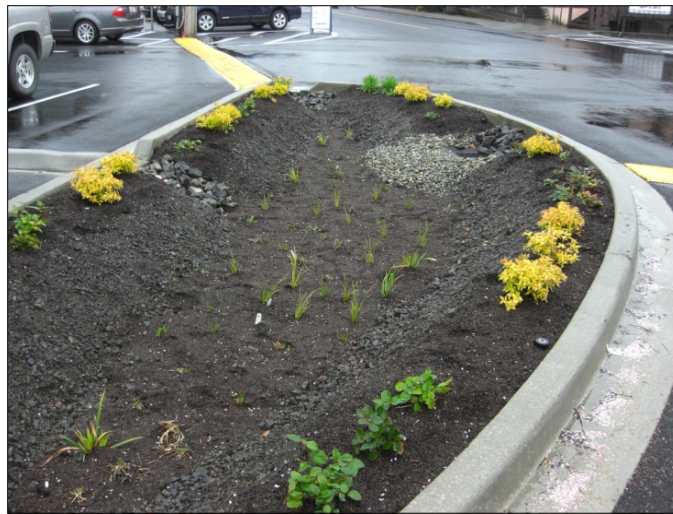
Figure 32. Newly-constructed Anderson Parkway bioretention cell with immature plantings.
