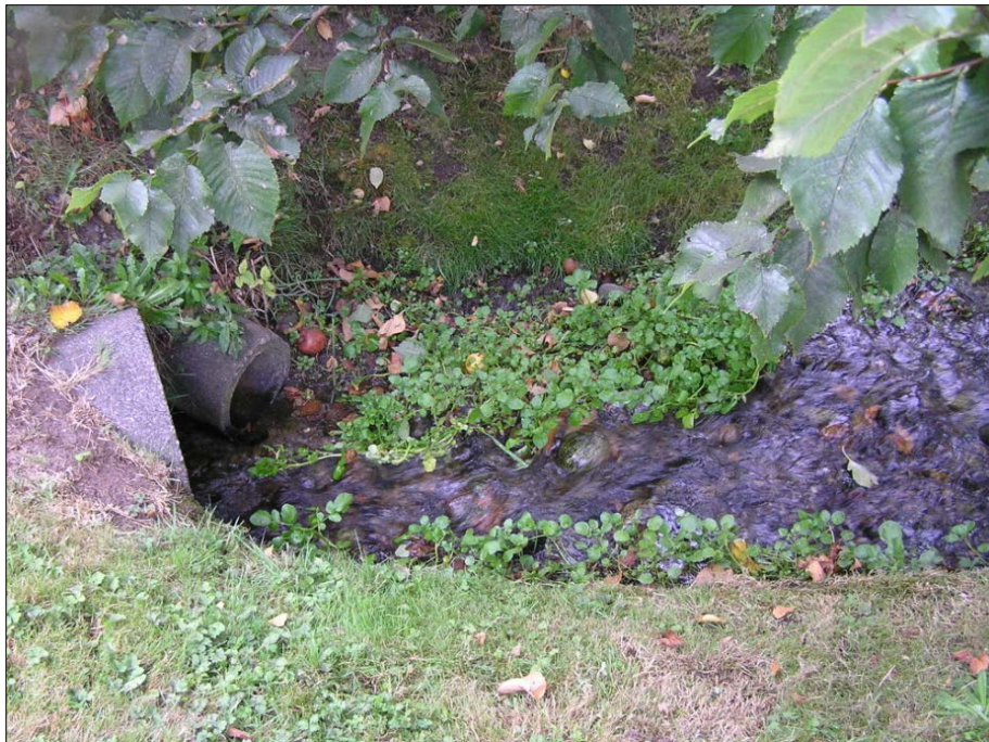
Figure 36. Poulsbo Creek, a perennial stream that discharges via an outfall to Liberty Bay, is piped in some areas of Poulsbo and open in others.
