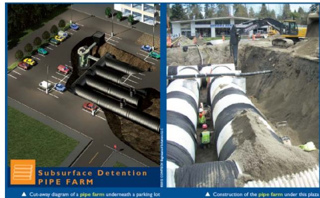
Stormwater flows into large pipes installed under the parking lot where it is stored and then slowly released. This helps reduce downstream flooding and erosion in Echo Lake, Lake Ballinger and McAleer Creek.
