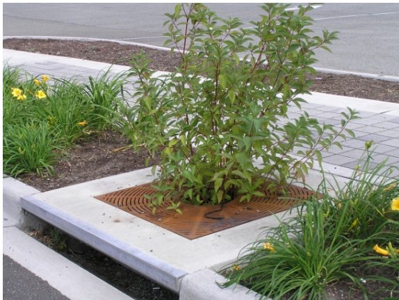
The city installed 17 Filterra* stormwater treatment units, also known as bioretention boxes.
