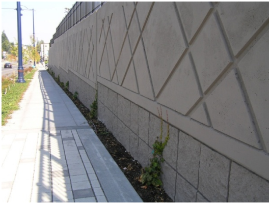
Pervious paver walkways and “green walls”
