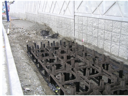
Under the walkways, modular root boxes hold lightly compacted soils in place, which supports the sidewalks and provides space for healthy root and tree growth.
