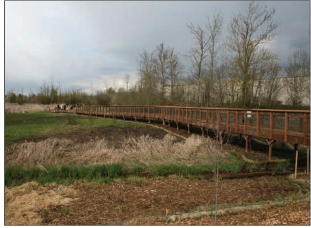
FIGURE 4.8.4 - FOOTBRIDGE WITH MINIMAL EXCAVATION FOUNDATION Completed foot-bridge utilizing minimal excavation foundations at the Auburn Environmental Park in Auburn, Washington. Source: AHBL, Inc.
