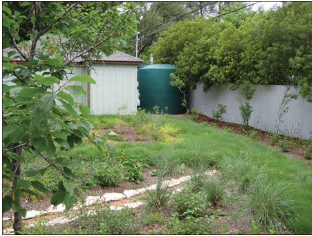
FIGURE 4.9.1 - POLYETHYLENE CISTERN Polyethylene cistern used to meet residential non-potable water demand. Source: Innovative Water Systems, LLC
