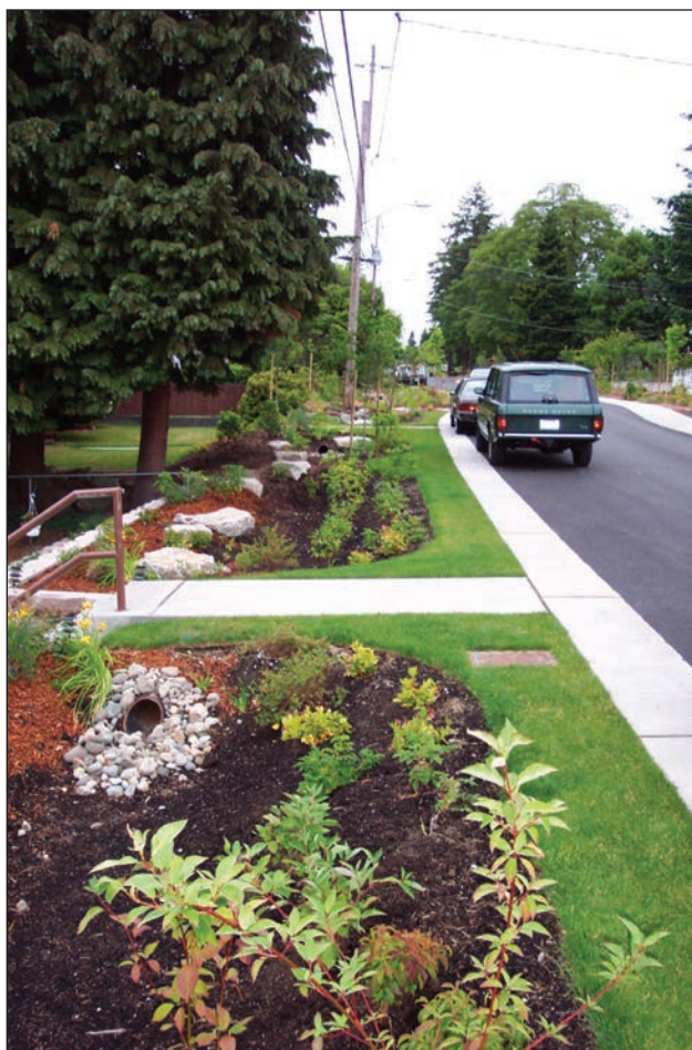
FIGURE 4.4.12 Bioretention area with flush curb and shoulder. Source: Photo by Curtis Hinman
