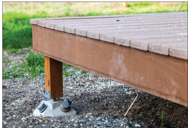
FIGURE 4.8.2 - USE OF MINIMAL EXCAVATION FOUNDATIONS FOR ACCESSORY STRUCTURES Deck constructed over piers. Source: City of Spokane
