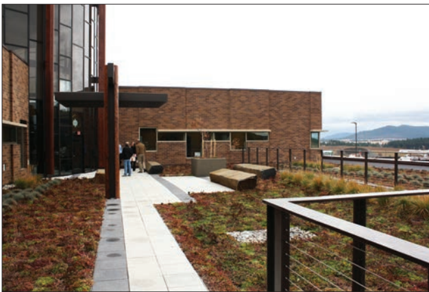
FIGURE 4.7.2 - VEGETATED ROOF – INTENSIVE DESIGN Bewewah Medical Center, Plummer ID, Intensive vegetated roof. Source: NAC Architecture
