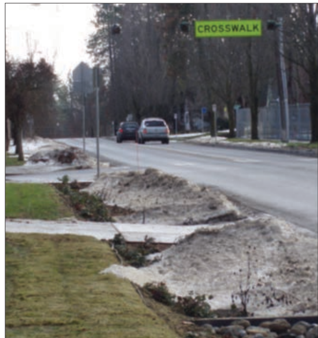
FIGURE 3.2 BIORETENTION SNOW STORAGE Snow storage in roadside bioretention in Spokane Source: AHBL, Inc. courtesy of Yakima Regional Low Impact Development Stormwater Design Manual
