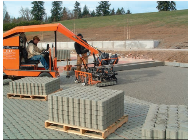
FIGURE 4.6.11 Mechanical paver installation. Source: Curtis Hinman
