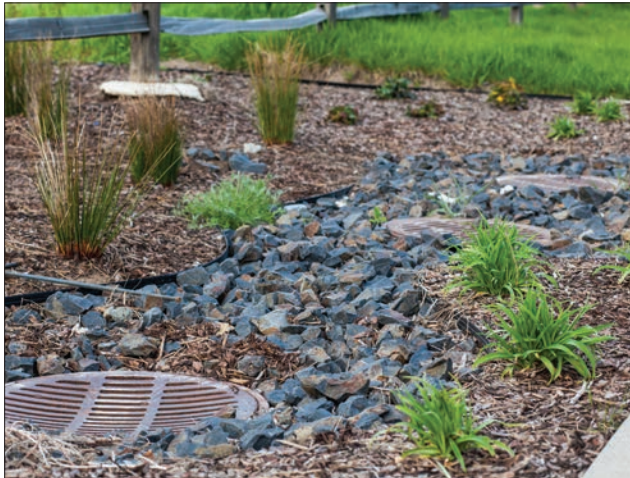
FIGURE 4.4.3 Arid climate bioretention example, Spokane. Source: City of Spokane
