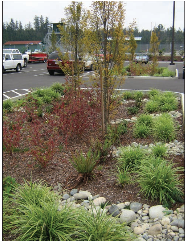
FIGURE 3.10 PARKING LOT BIORETENTION Bioretention integrated into required parking lot landscaping Source: AHBL, Inc.
