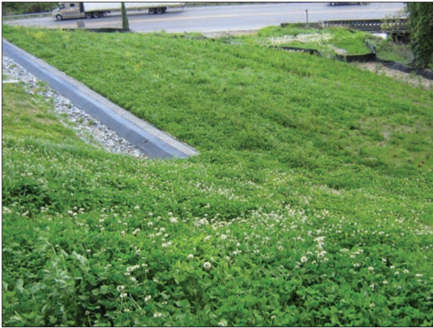
FIGURE 4.3.1 Engineered dispersion with level spreader Source: AHBL, Inc.
