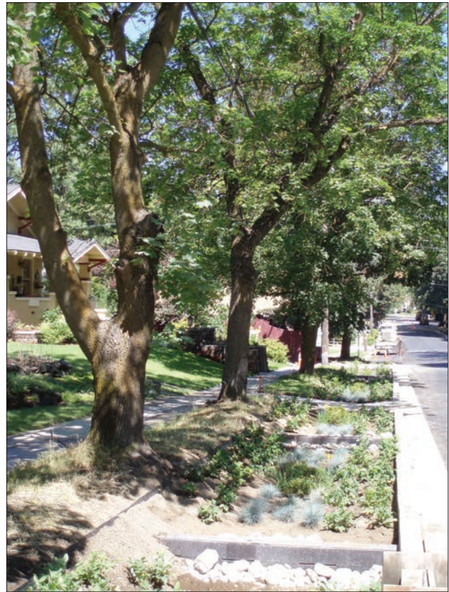
FIGURE 4.5.2 A bioretention facility utilizing existing mature street trees. Source: AHBL, Inc.
