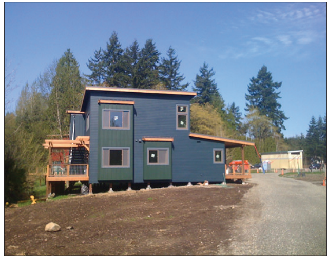
FIGURE 4.8.1 - USE OF MINIMAL EXCAVATION FOUNDATIONS FOR RESIDENTIAL DWELLING Single-family dwelling unit constructed over piers. Source: Photo with permission of Pin Foundations, Inc.
