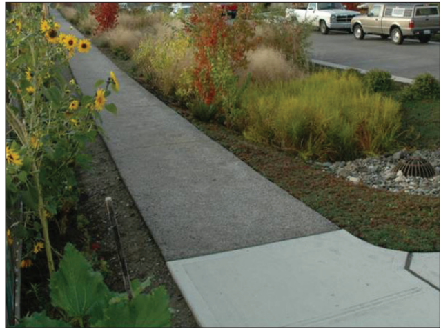
FIGURE 4.6.7 Pervious concrete. Source: HDR Engineering
