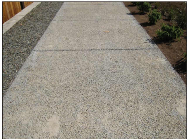
FIGURE 4.6.1 Permeable pavement. Source: HDR Engineering
