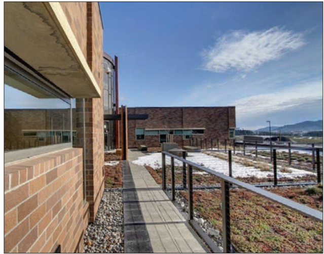
FIGURE 3.12 VEGETATED ROOF Benewah Medical Wellness Center vegetated roof, Plummer, Idaho. Source: NAC Architecture
