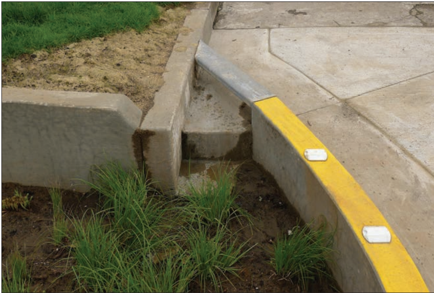
FIGURE 4.4.7 Curb cut inlet with drop to prevent clogging at flow entrance. Source: Photo by Curtis Hinman Illustration courtesy of the Bureau of Environmental Services, City of Portland, OR.
