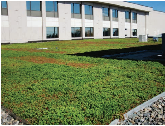
FIGURE 4.7.1 - VEGETATED ROOF – EXTENSIVE DESIGN St Mary Medical Center, Walla Walla, extensive vegetated roof. Source: Xero Flor America (XFA) and Tremco
