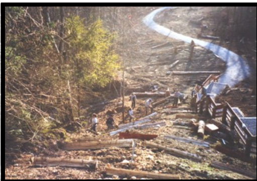
Heart Attack Hill, Post Fire, Pre-Restoration.
