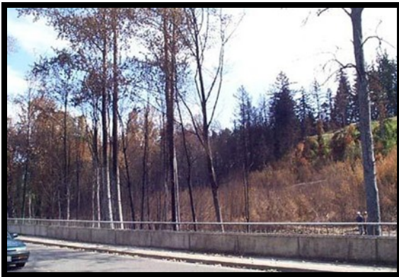
Boulder Bend, Post Fire, Pre-Restoration.
