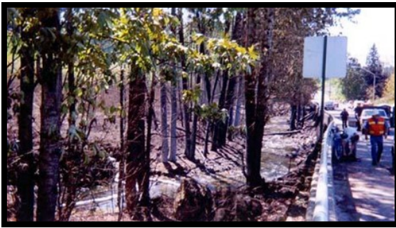
Boulder Bend, Post Fire, Pre-Restoration.
