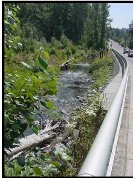
Boulder Bend, Post Restoration.
