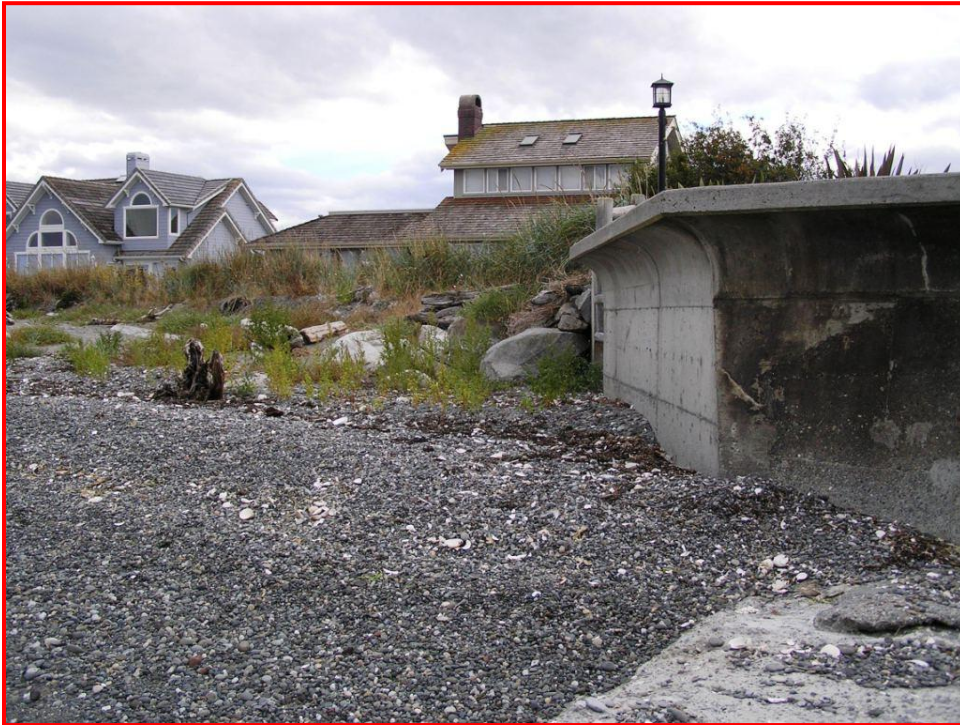
Figure 12: End erosion effects caused by this seawall resulted in the need for hard rock on the adjacent neighboring property. (Kelsey Gianou photo.)
