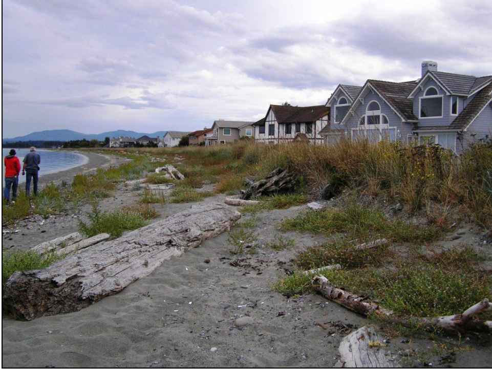
Figure 19: Seashore Lane after soft shoreline stabilization.
