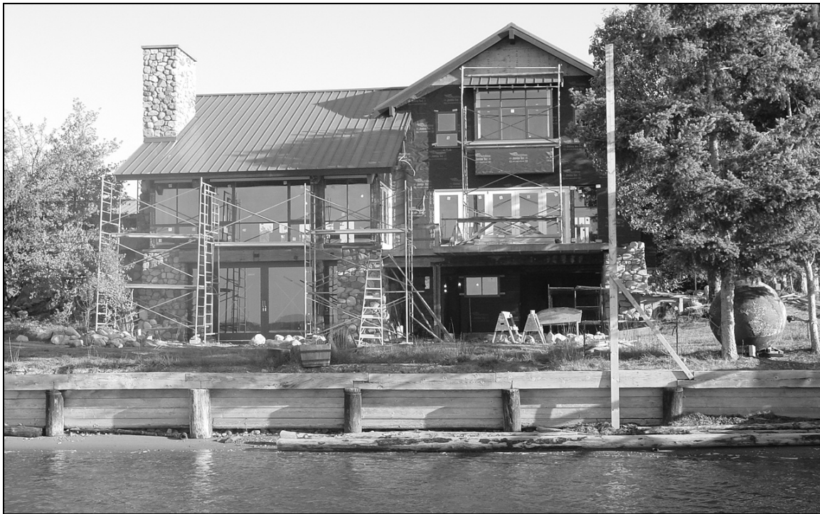
Figure 28: Fisherman's Bay, Lopez Island, before bulkhead removal.
