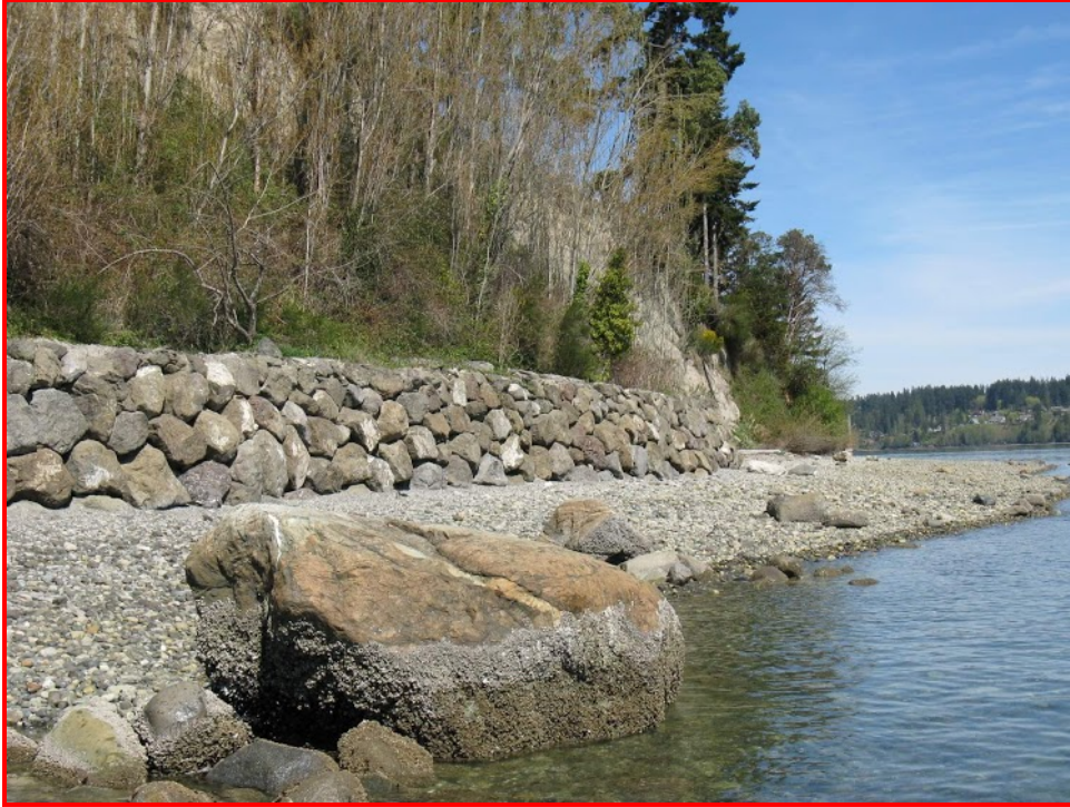
Figure 8: This rock seawall prevents erosion and the delivery of sediment to the beach. (Hugh Shipman photo.)
