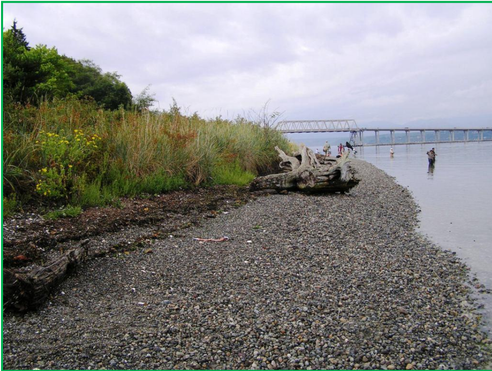
Figure 14: Enhanced aquatic-terrestrial connectivity and backshore habitat. This soft shoreline stabilization project replaced original riprap armoring. (Kelsey Gianou photo.)
