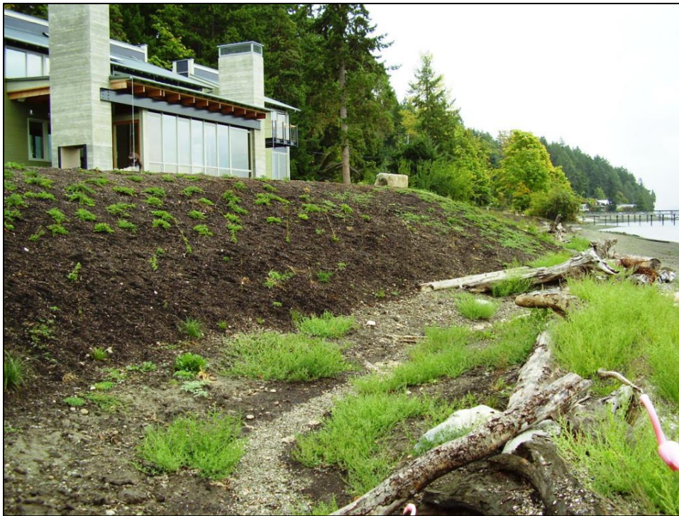
Figure 22: Port Blakely Harbor, Bainbridge Island, after stabilization.
