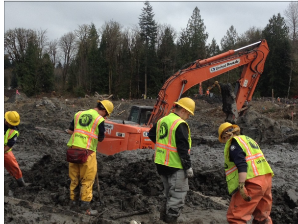
WCC crew members dig trenches at the debris field.
