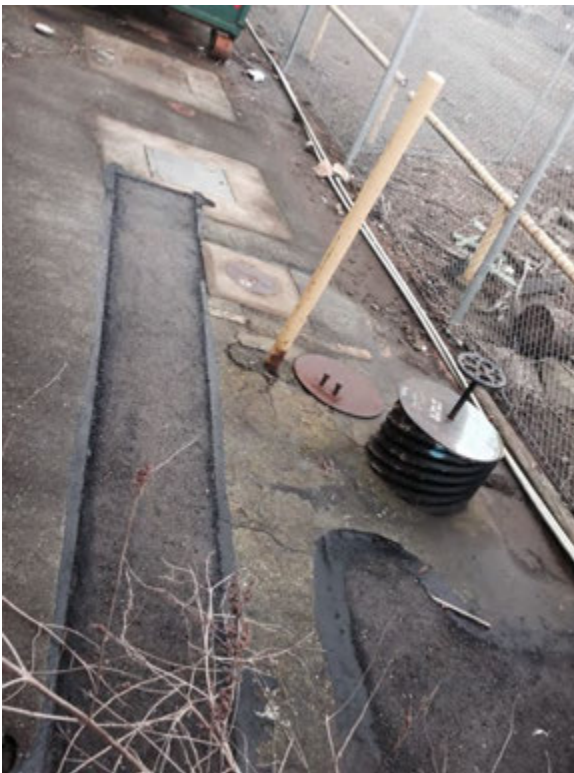
Photo 6. BP Terminal showing Compliance Monitoring Well AMW-01 to the left and behind the yellow bollard. Additionally, Recovery Well RW-10 is located directly behind AMW-01. Recovery Well RW-10 is an active pumping well utilized as part of the Groundwater/LNAPL Recovery System. Well heads are flush mounted to ground surface.
