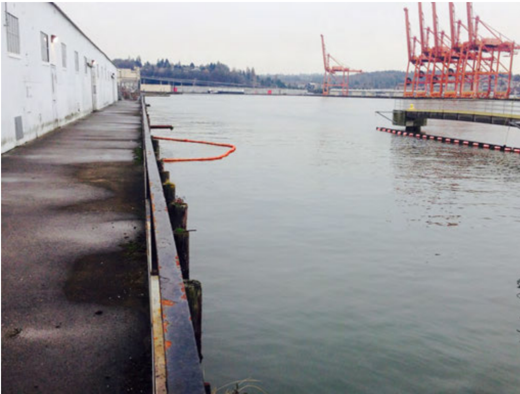
Photo 5. BP Terminal looking south along the seawall and West Waterway with orange boom to capture any sheen or floating product on waterway as a safety measure. Along this walkway are near shore compliance monitoring wells to evaluate current conditions and protect waterway. Well heads not easily visible.
