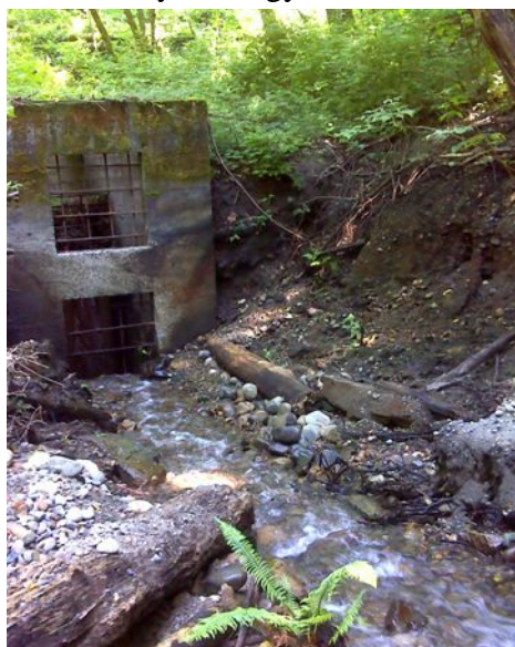
Figure 3. Sediment Retention to Address Bank Erosion, Rody Creek
