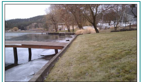
The failing bulkhead prior to removal
