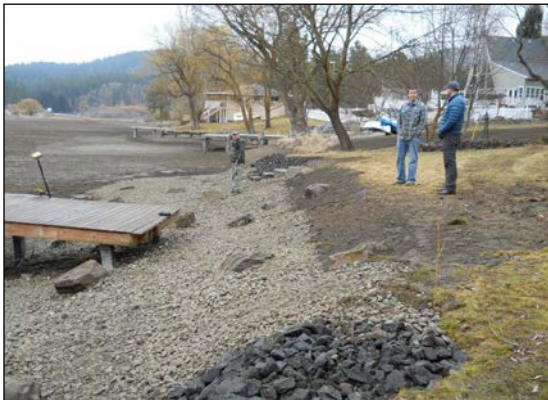
The Staggs' shoreline after completed construction
