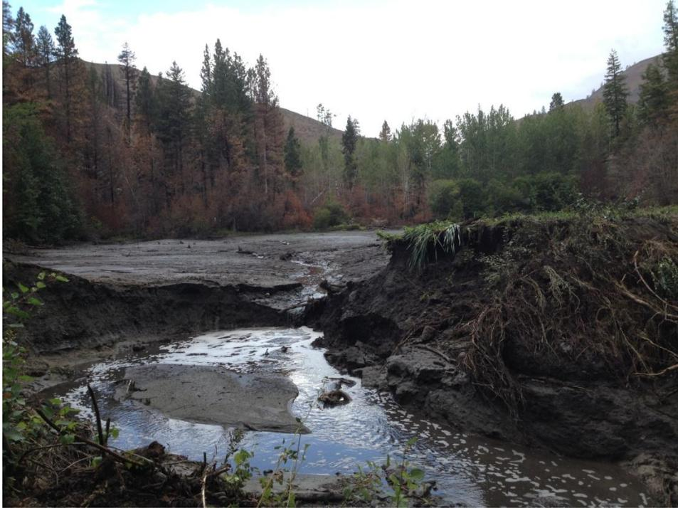
3. Wenner Lake No.2 eroded spillway on Aug 24<sup>th</sup>, looking upstream (north).
