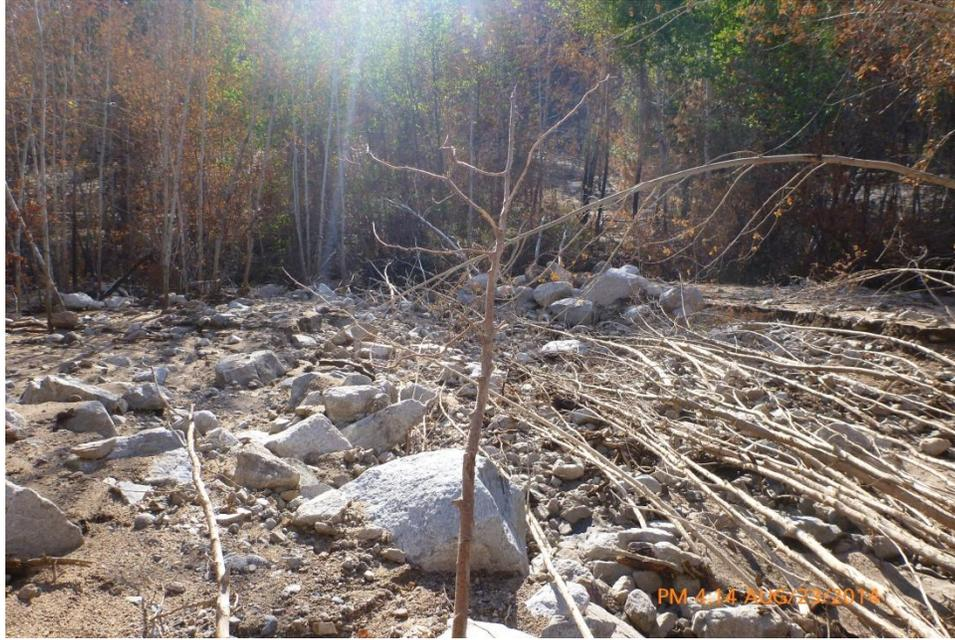
7. Rabel Dam (Wenner Lake No.4) existing spillway on Aug 23<sup>rd</sup>, blocked by debris flow, looking downstream (south).
