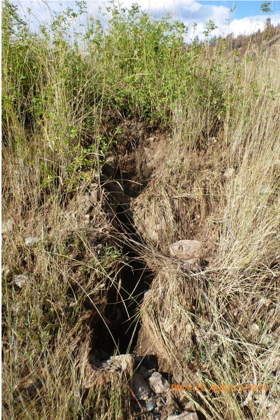
9. Rabel Dam (Wenner Lake No.4) downstream face on Aug 23<sup>rd</sup>, small erosion gully from overtopping flows; looking upstream (north).
