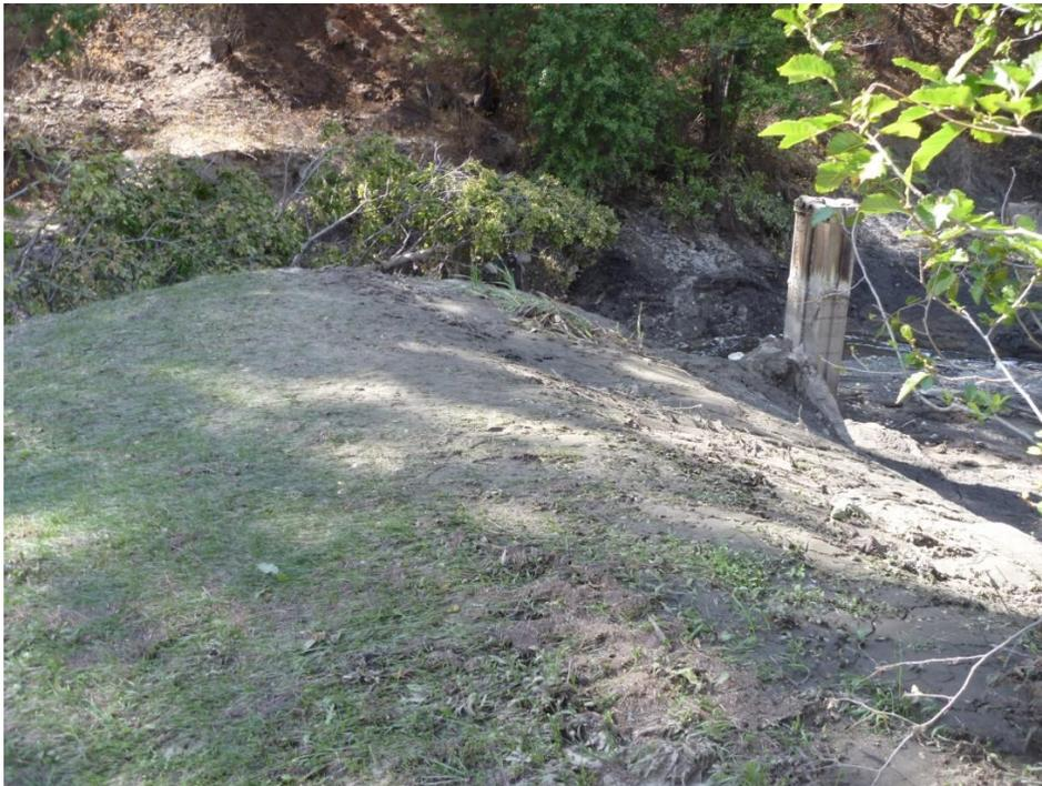
6. Wenner Lake No.3 dam and eroded spillway on Aug 27<sup>th</sup>, looking right (west).
