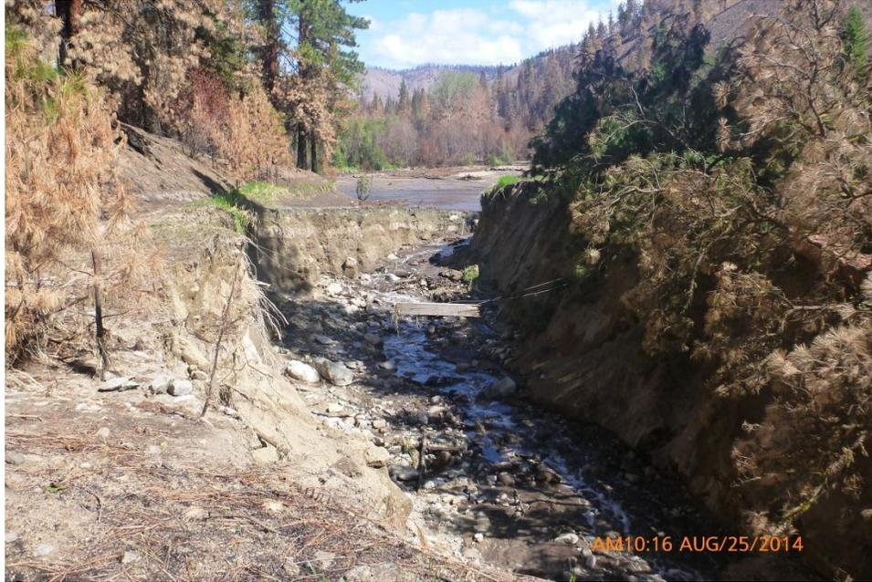
14. Hawkins Dam (Wenner Lake No.5) eroded spillway on Aug 25<sup>th</sup>, looking upstream (north).
