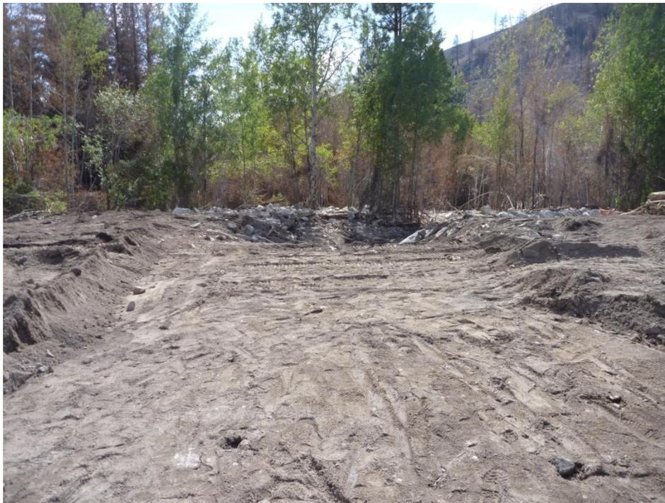
11. Rabel Dam (Wenner Lake No.4) new spillway on Aug 27<sup>th</sup>, high-flow channel to right of pilot channel; looking downstream (south).
