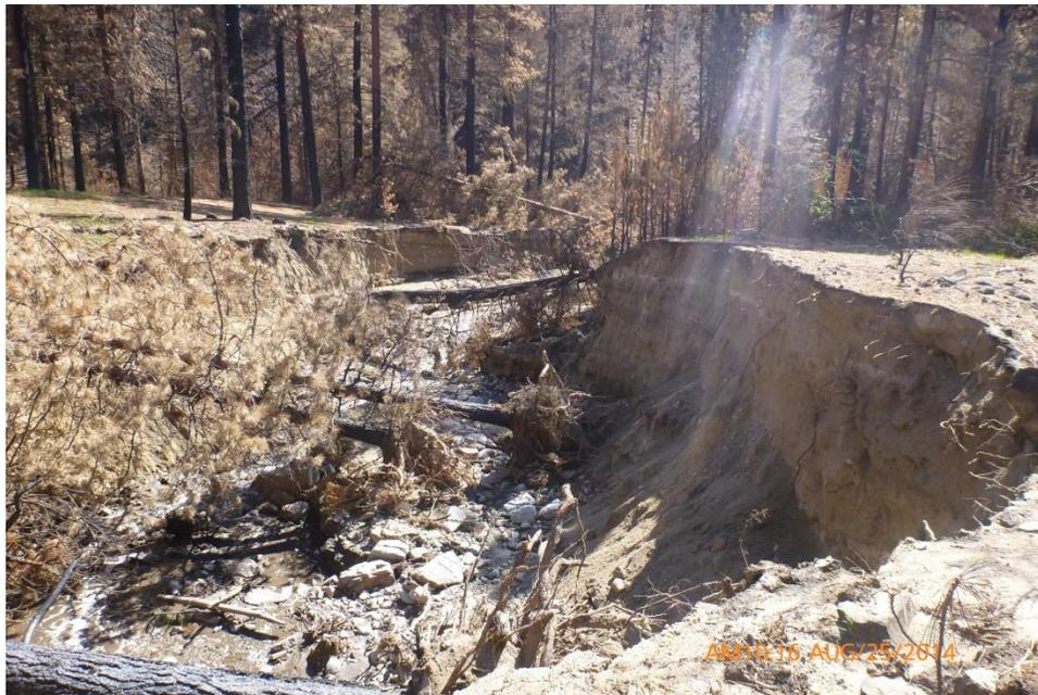
15. Hawkins Dam (Wenner Lake No.5) eroded spillway on Aug 25<sup>th</sup>, looking downstream (south).
