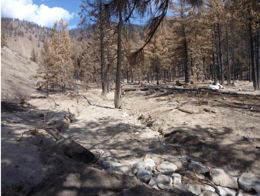
12. Rabel Dam (Wenner Lake No.4) on Aug 27<sup>th</sup>, valley at left abutment, source of debris flow that blocked the spillway; looking east. At the large trees, sediment is 5 feet thick.
