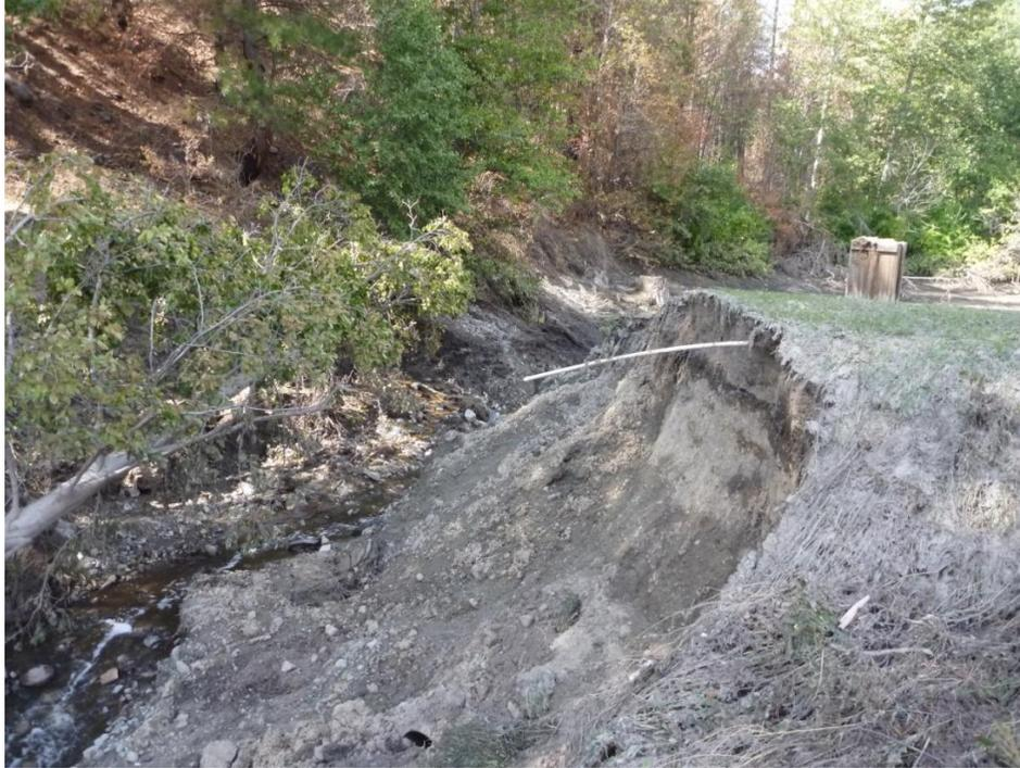
5. Wenner Lake No.3 eroded spillway on Aug 27<sup>th</sup>, looking upstream (north).
