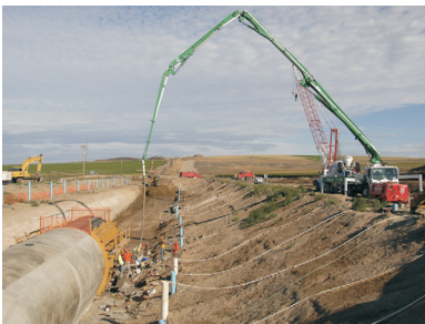
Expanded infrastructure will provide replacement surface water for up to 90,000 acres currently irrigated by groundwater from the declining aquifer of the Odessa Subarea.
