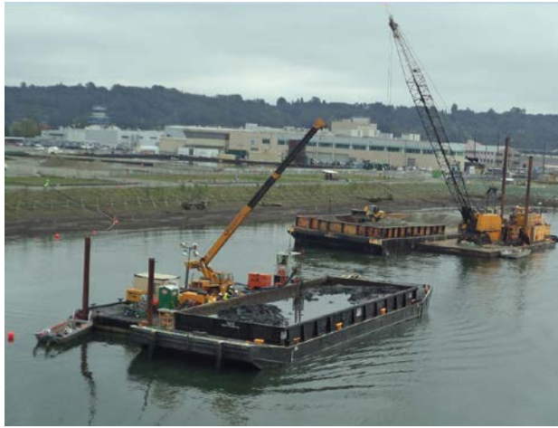
Lower Duwamish dredging and restoration work at a site in Seattle.
