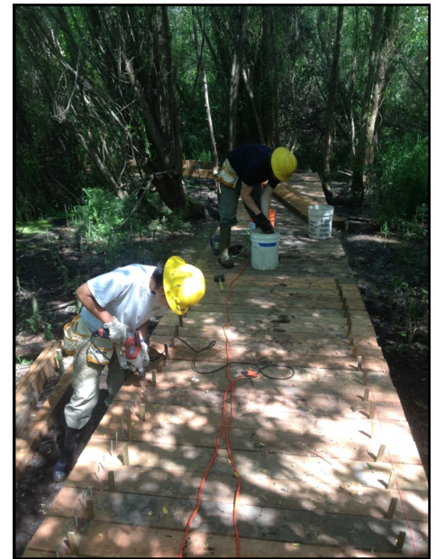
Above Left: Section of boardwalk that has had cedar planks laid by hand.
