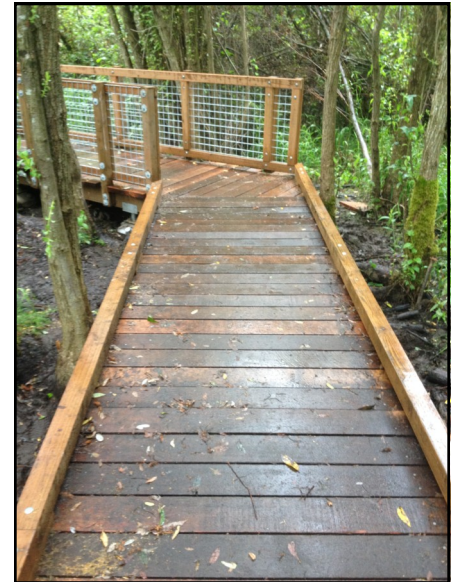
The completed boardwalk is ADA accessible and fun for all ages!
