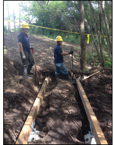
Above: Brackets are in place to hold wood support beams.
