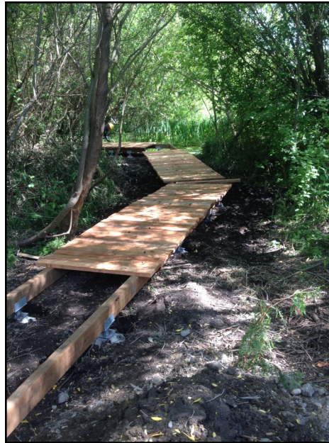
Above Left: Section of boardwalk that has had cedar planks laid by hand.
