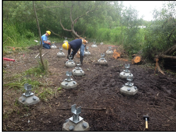
Above: Brackets are in place to hold wood support beams.
