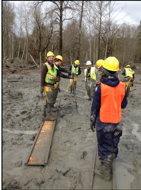
Balancing on I-beams while working in debris field
