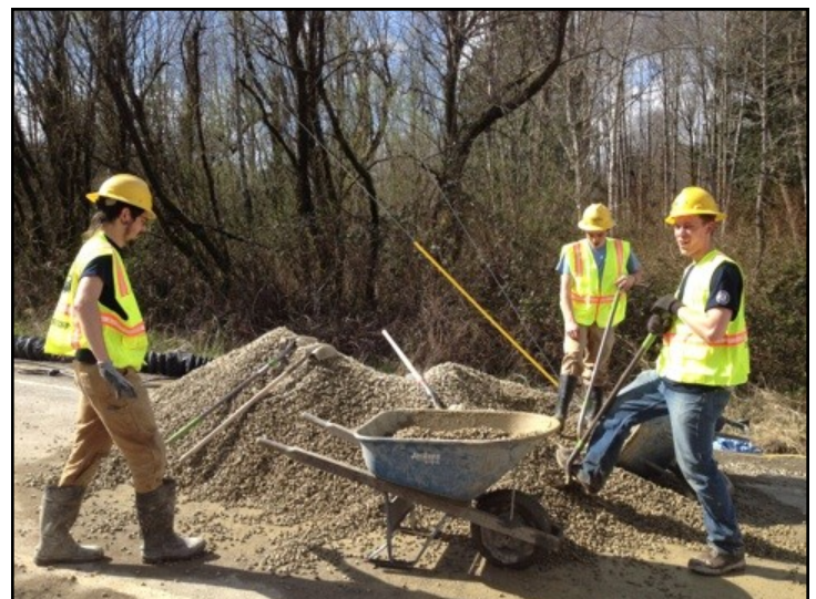
Moving and spreading gravel all around the base camps
