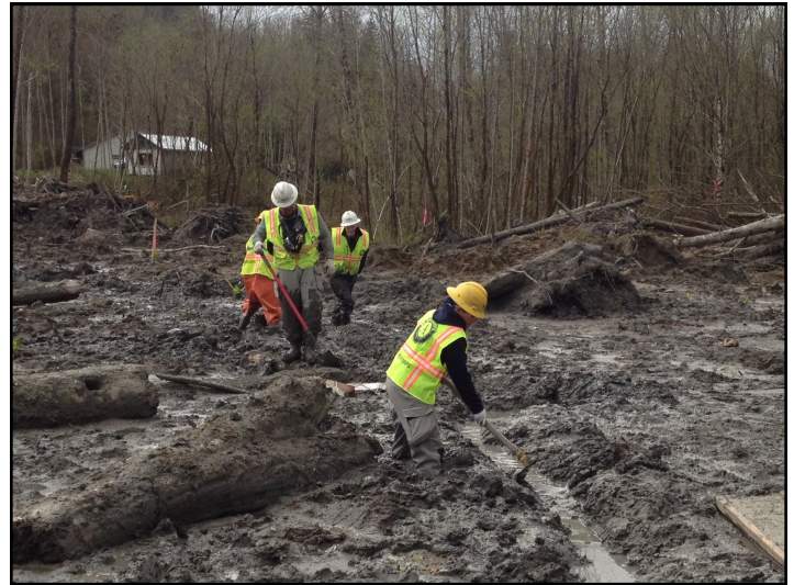
Digging trenches to dewater the debris field
