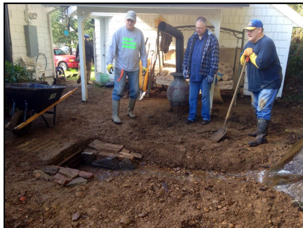
Hardworking volunteers admire a new brick wall to guide the stream.
