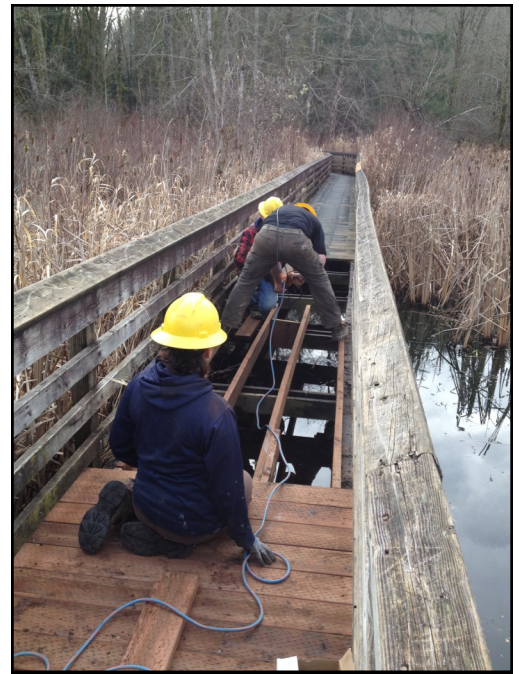
1. Demo and rebuild old boardwalk so that it can support the weight of a quad and a trailer of gravel. Don't lose any measuring tapes in the water.
