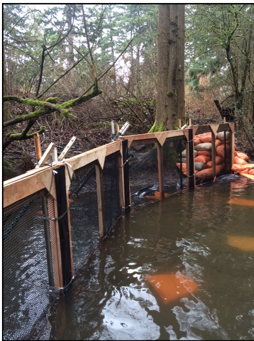
Weir panels funnel fish to trap.
