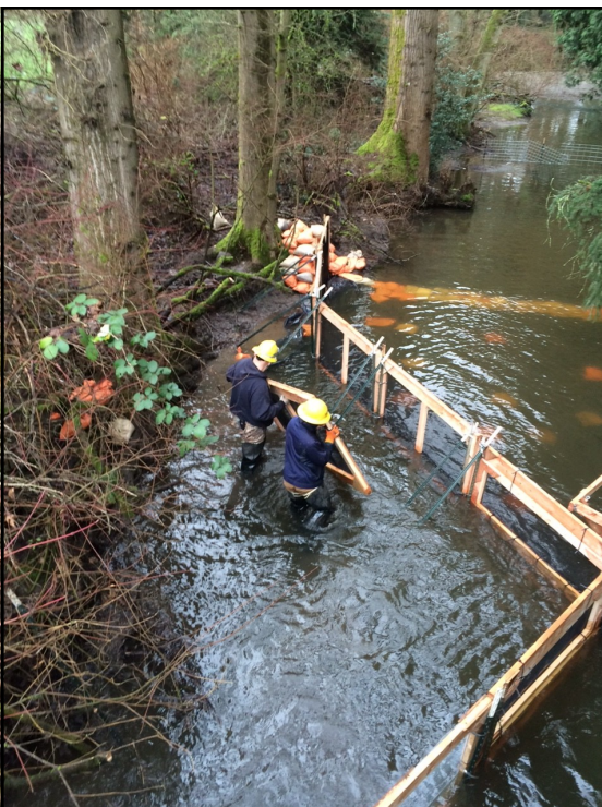
Moving weir panels into place.
