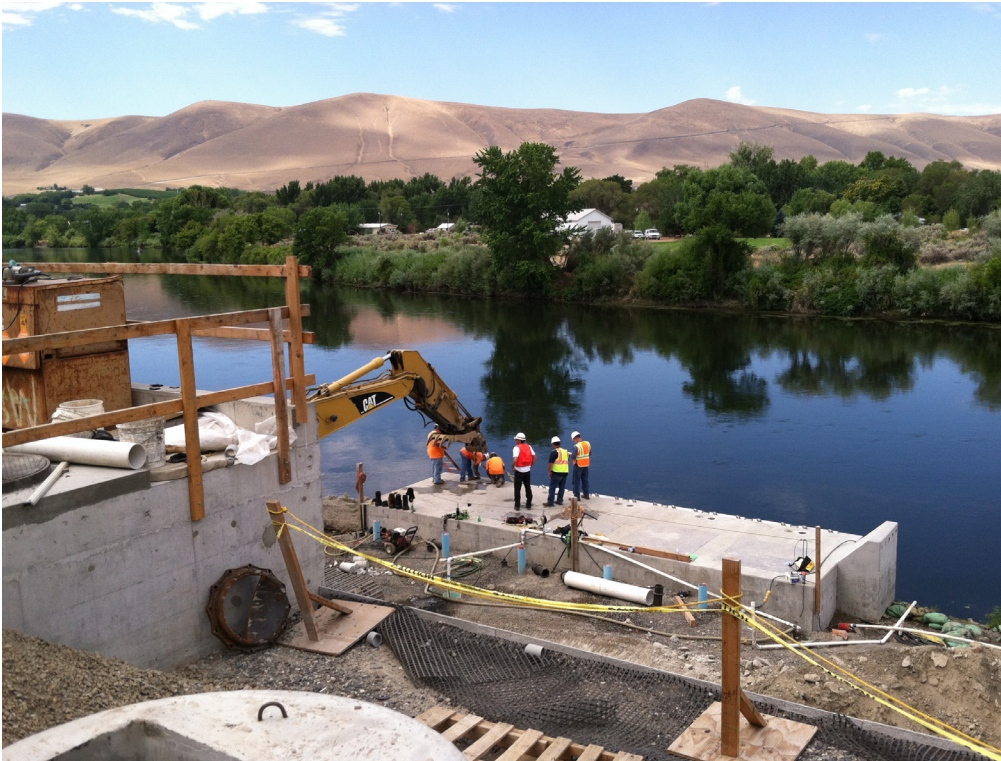
A newly constructed diversion at Kiona allows KID to deliver water to satisfy the irrigation of 1,785 acres on Red Mountain, funded in part by OCR.
