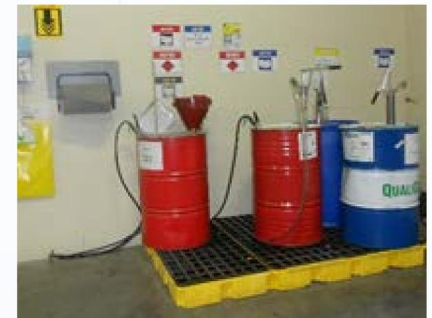
*After: Barrels are labeled and secondary containment is installed underneath.*
