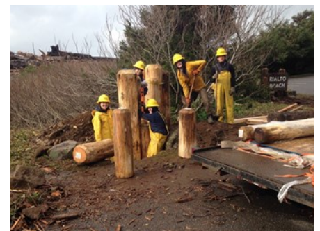
Installing the sign support logs.
