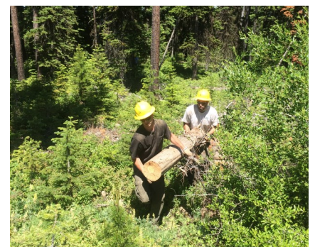
Josh Knight and Hayden Lucia hauling construction materials from the forest. Photo submitted by Adam Hein.
