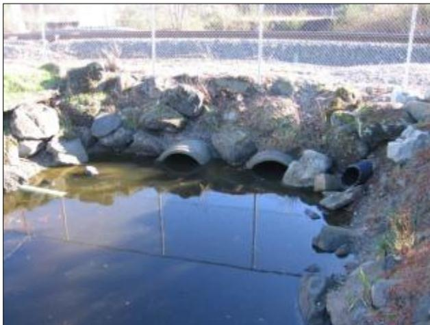
**Figure 6-11: Culverts under BNSF rail line in Edmonds. Salish Sea tidal influence extends under the BNSF line into Edmonds Marsh.**
