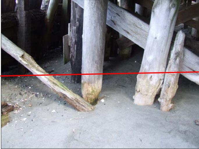
**Figure 4-39: Staining and deterioration of wood support pilings under a cabin on the beach.**
