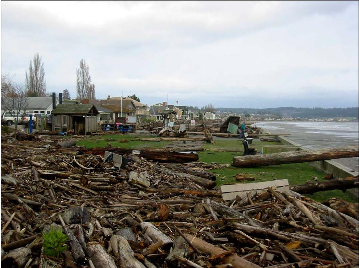
**Figure 4-6: Aftermath of an extreme high water event; OHWM located at the waterward face of the bulkhead. Double Bluff Park, Whidbey Island – February 4, 2006. Photo courtesy of Hugh Shipman.**
