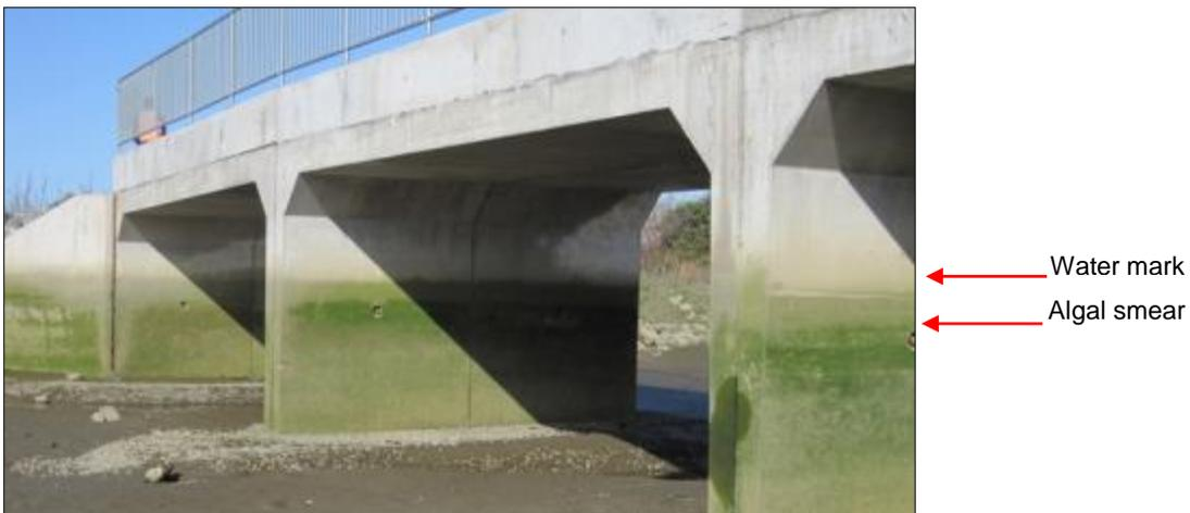
Figure 4-32: Algal smears on a concrete bridge in the lower Snohomish estuary.
