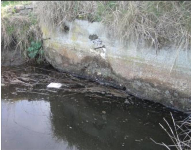
**Figure 4-38:** Water stains on a concrete wall in an estuary on Whidbey Island. Note how the upper end of the stained area coincides with the eroded shoreline to the left.
