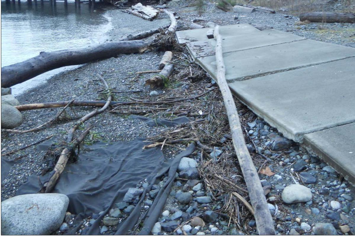
**Figure 4-22. Collapsed walkway undermined by waves, Port Gardner Bay. Note coarser substrate on the water side of walkway as wave deflection has eroded fines and gravel.**
