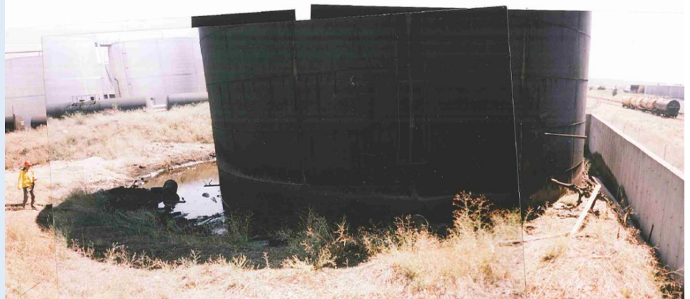
Figure 2. The BNSF Railway Black Tank around 1999. The tank stored petroleum products until 2006 when it was emptied and removed.
