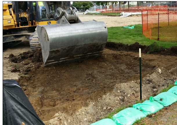
Contractors removed the top 12 inches of soil at Baltimore Park in Tacoma.
