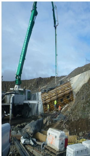
Construction at East Low Canal
