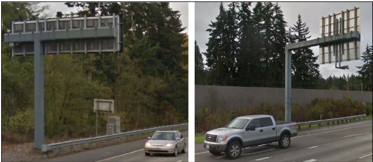
Figure M-3. Overhead highway signs.
