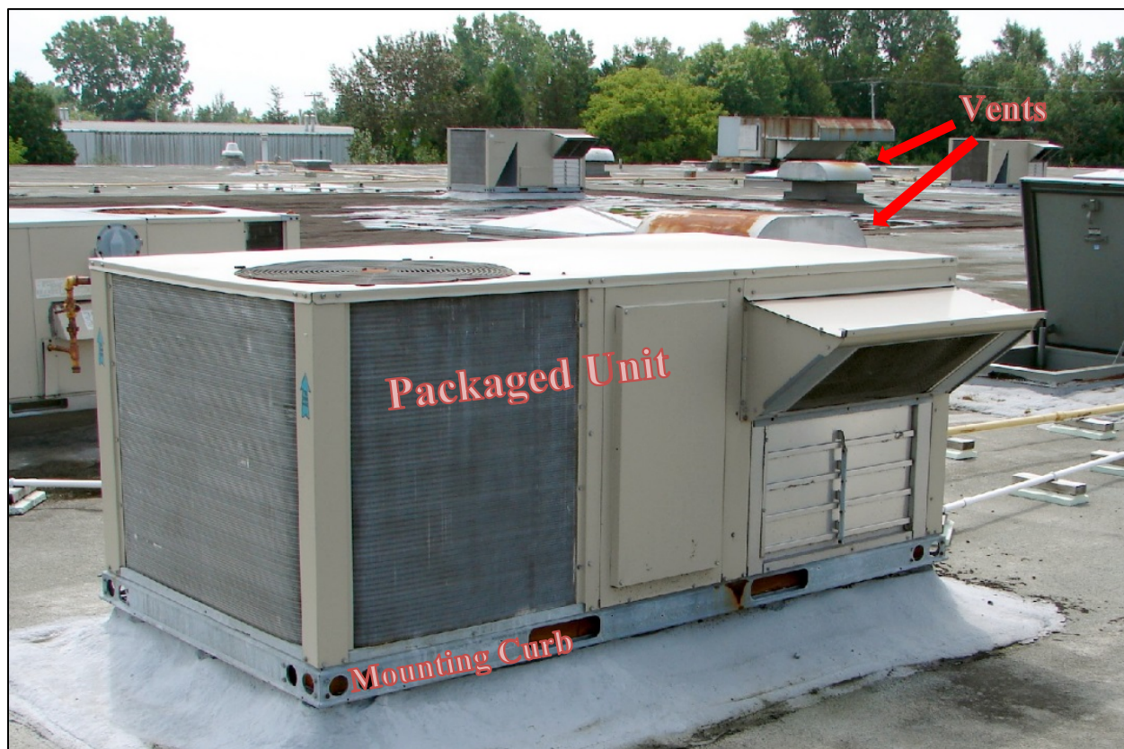
Figure I-1. Rooftop HVAC components including packaged unit, mounting curb, and vents
