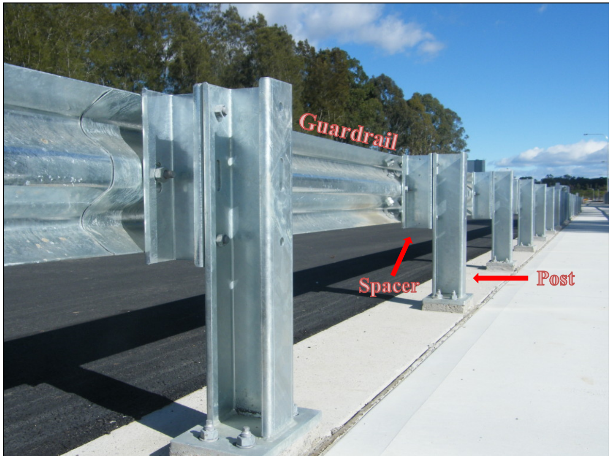
Figure K-1. Galvanized steel W-beam guardrail showing rail, posts, and spacers.
