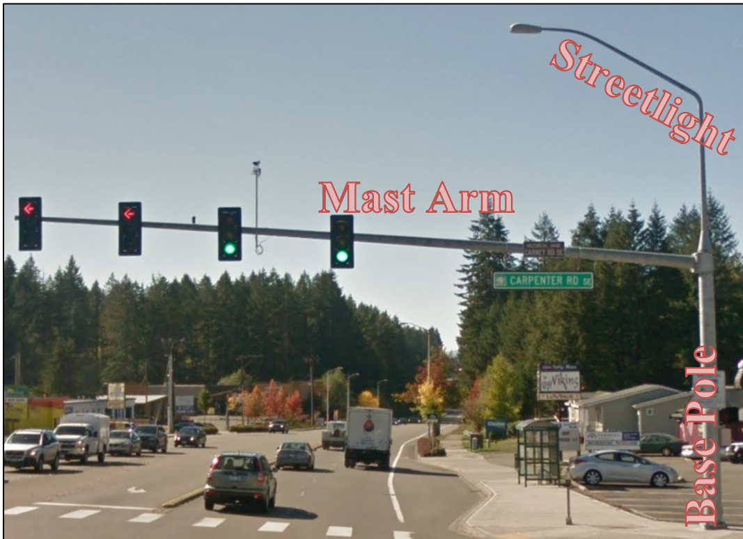
Figure L-2. Traffic signal with 40-foot streetlight controlling four lanes of traffic.
