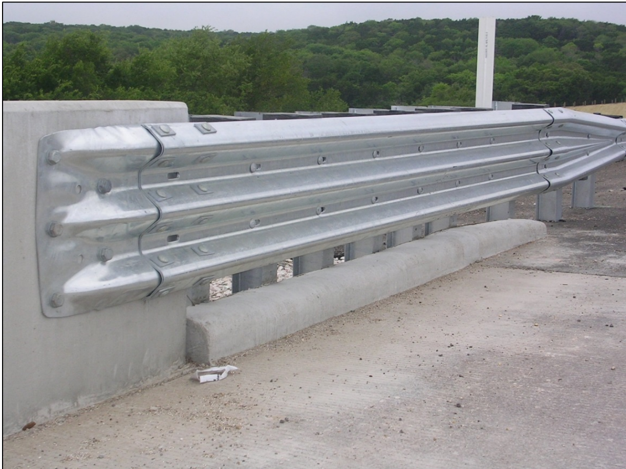
Figure K-2. Galvanized steel Thrie-beam guardrail showing transition section (upper right)
