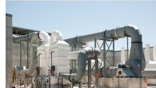
New odor control at a wastewater facility. Photo credit: LOTT Clean Water Alliance.
