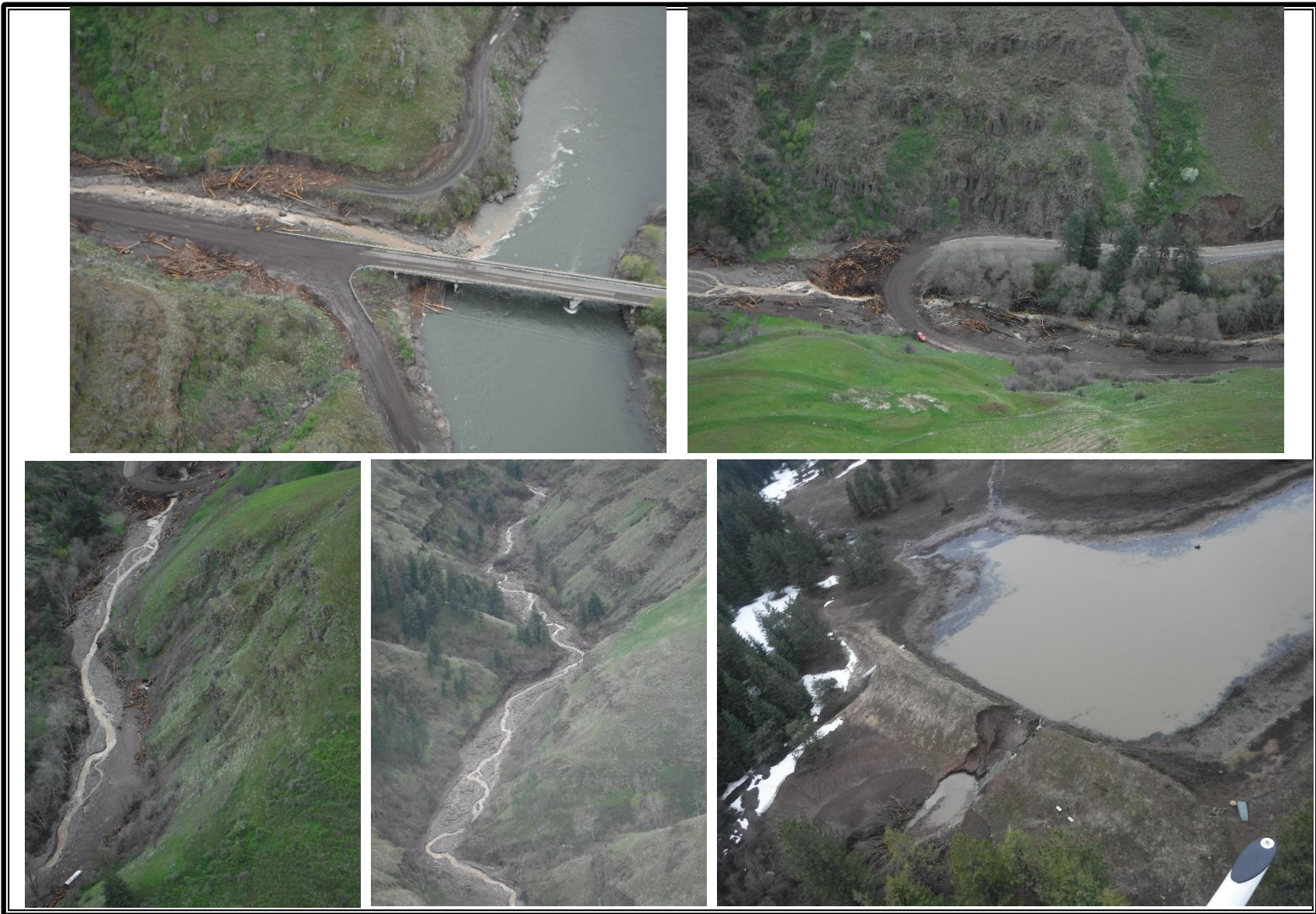
Figure 3. Remnants of the debris flow on Rattlesnake Creek and State Highway 129 from Bonasa Breaks Ranch Dam breach
