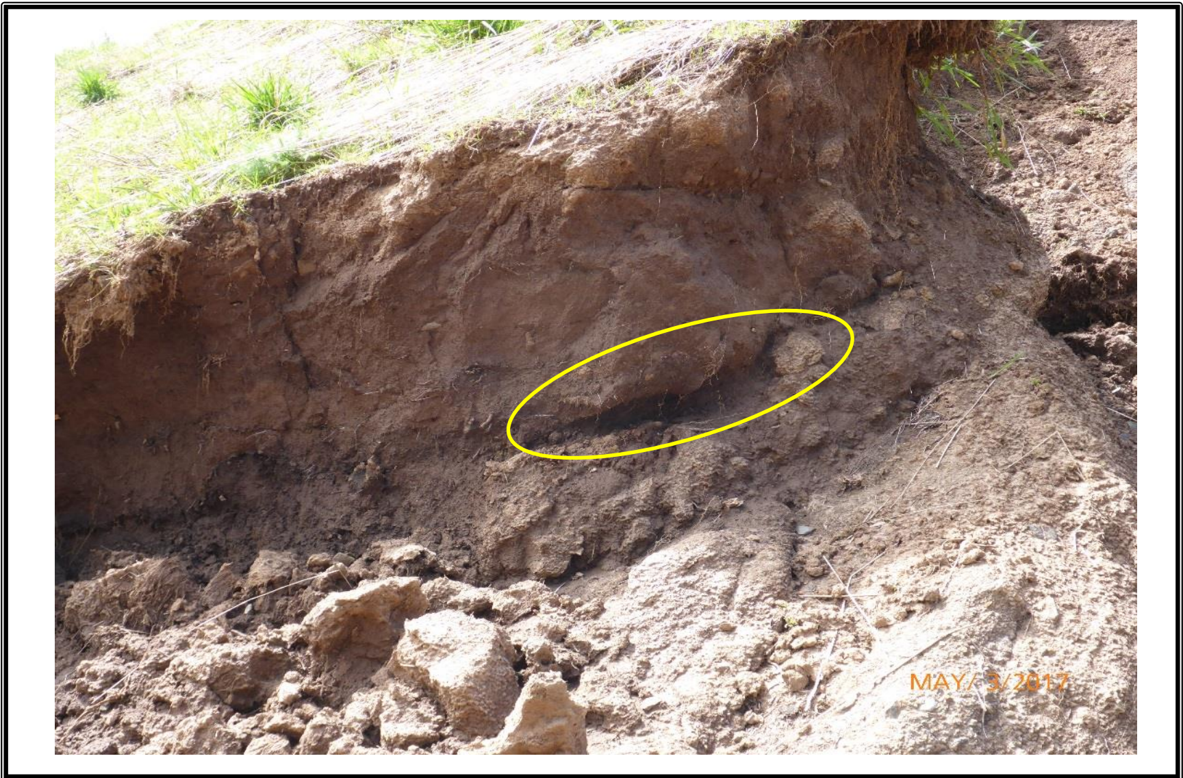
Figure 11. "Tube-like" feature on southern sidewall of breached section
