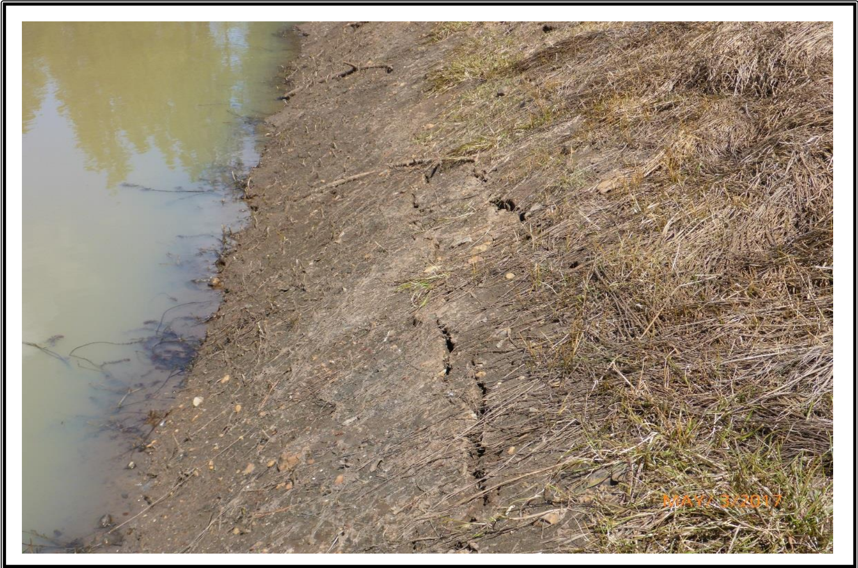
Figure 8. Bonasa Breaks Ranch breach: cracking on upstream slope along southern embankment section
