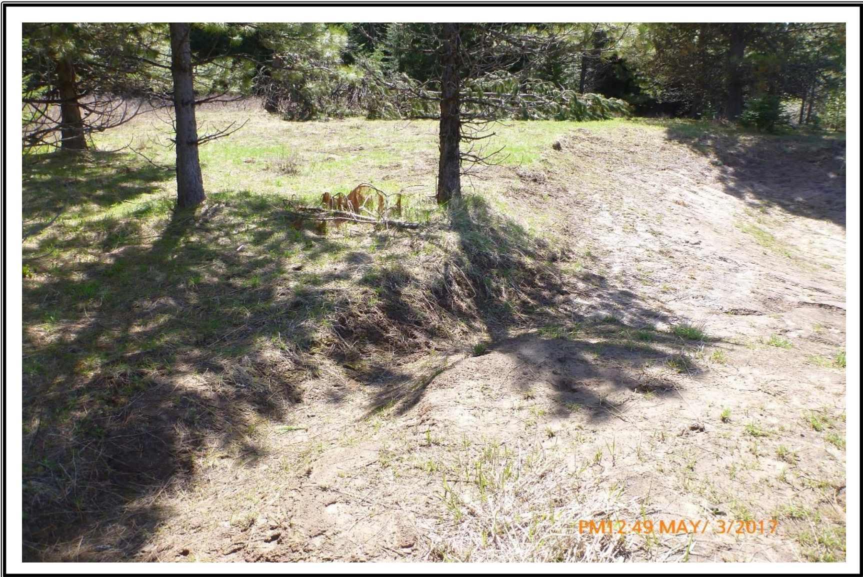
Figure 15. Channel on right abutment
