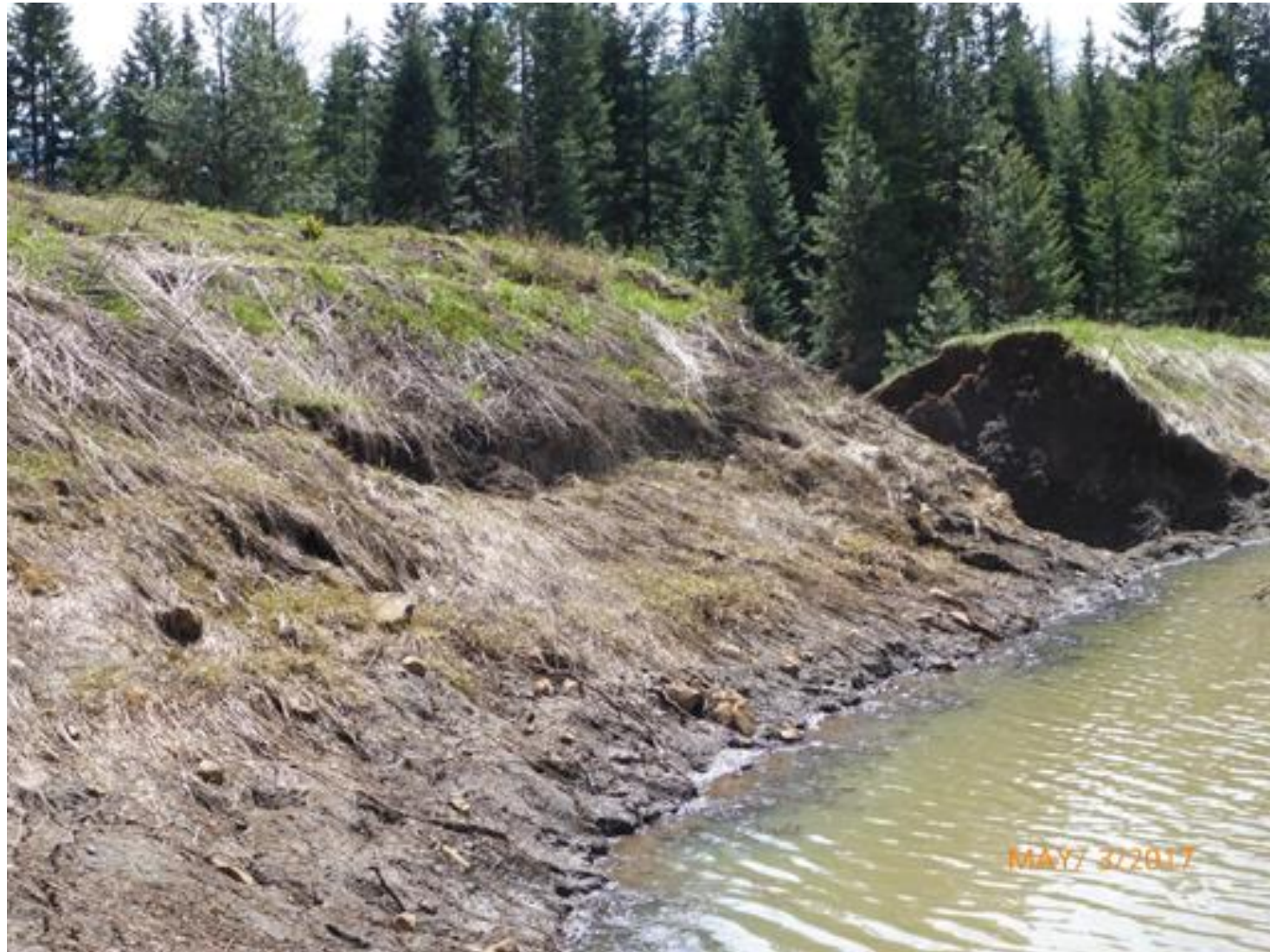
Figure 7. Bonasa Breaks Ranch Dam: soil movement likely induced by rapid drawdown failure on the upstream slope
