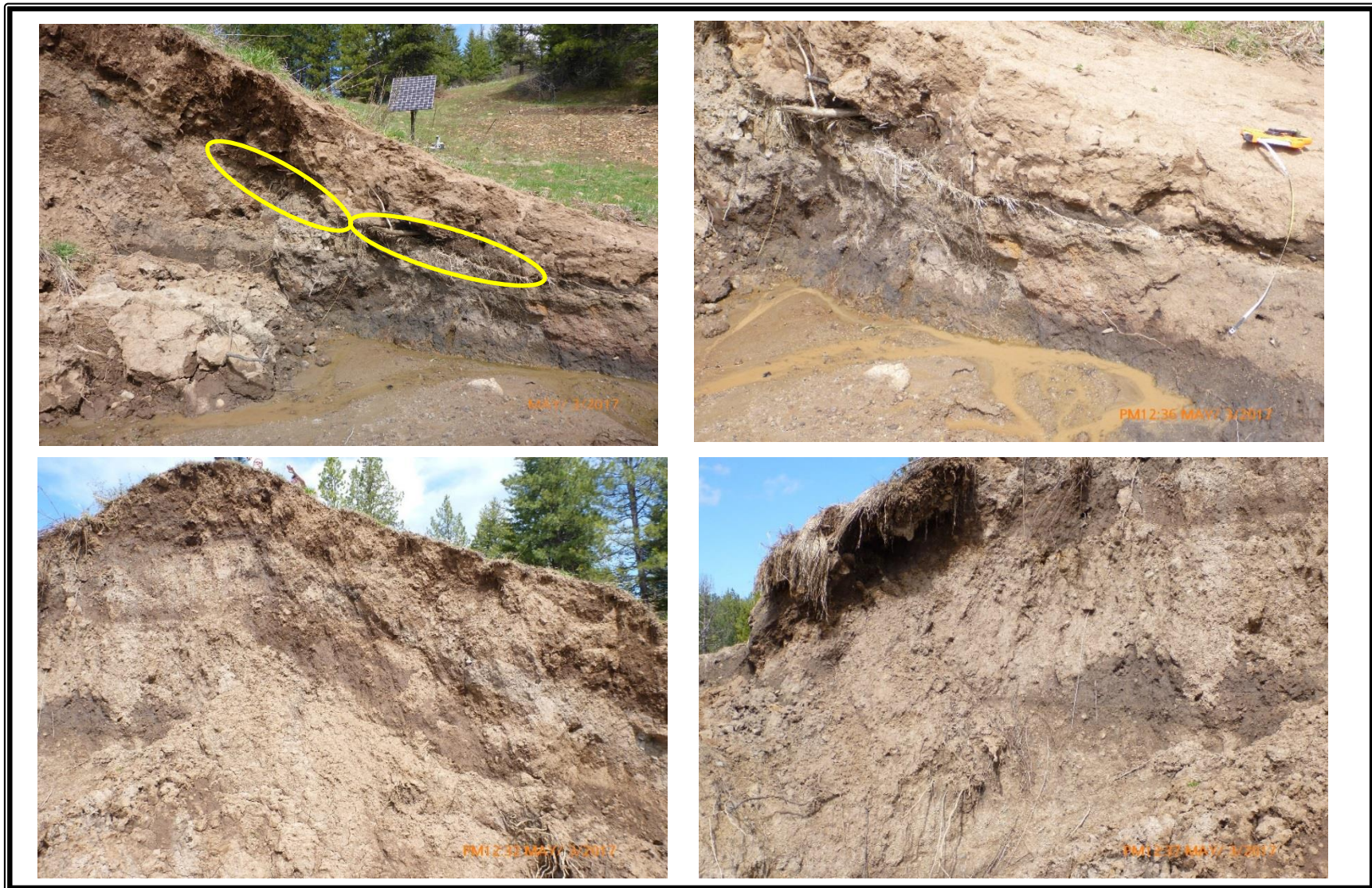
Figure 9. Bonasa Breaks Ranch downstream toe section. Notice the organic layer below the light brown top layer.
