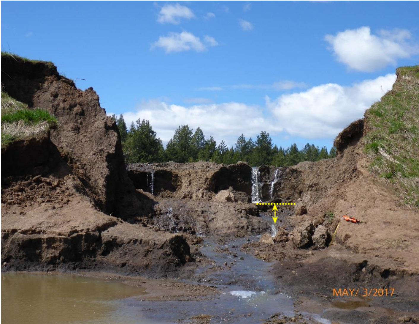
Figure 10. Bonasa Breaks Ranch breach section: Notice the difference in elevation at foundation level.
