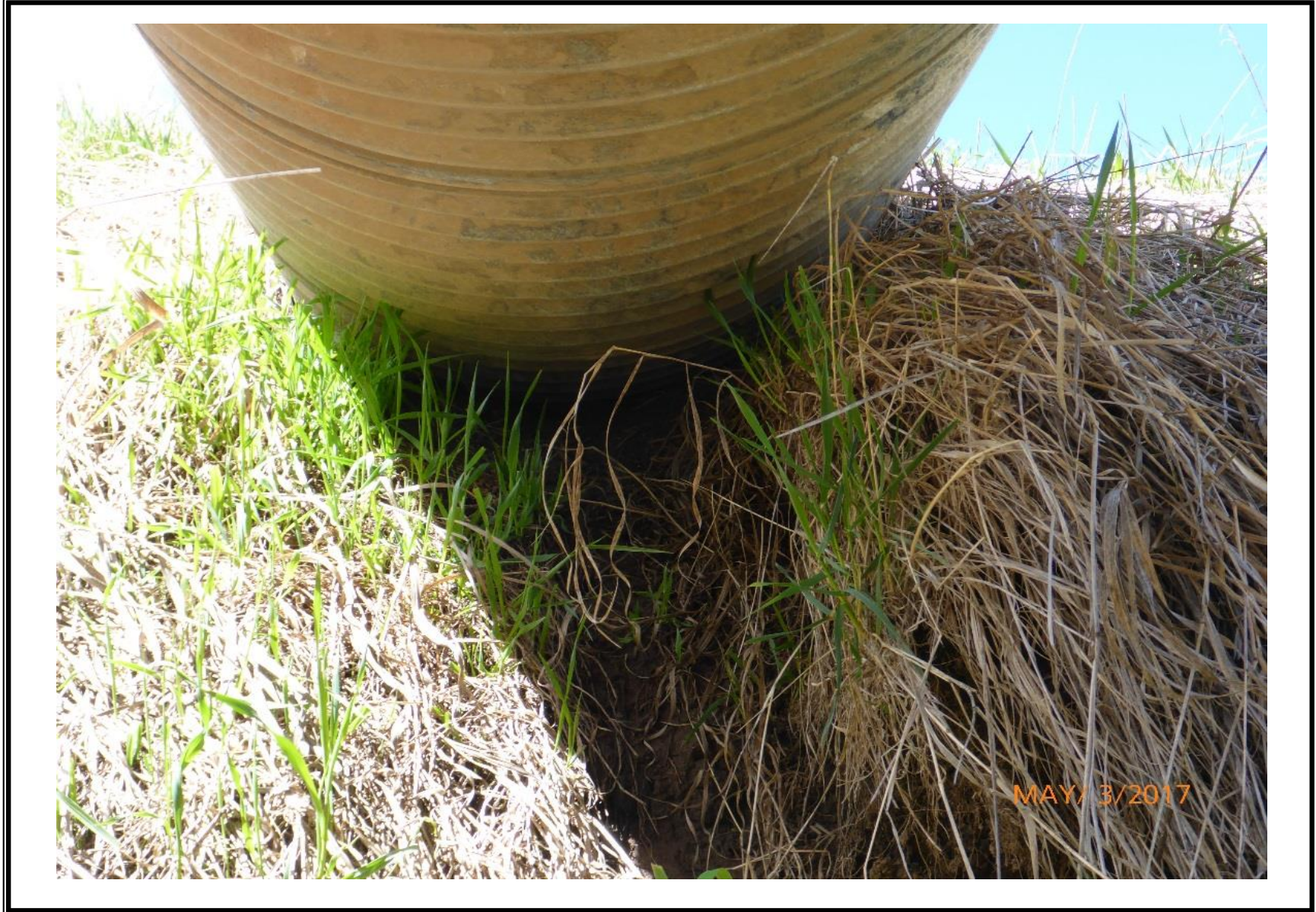
Figure 12. Downstream side of overflow conduit
