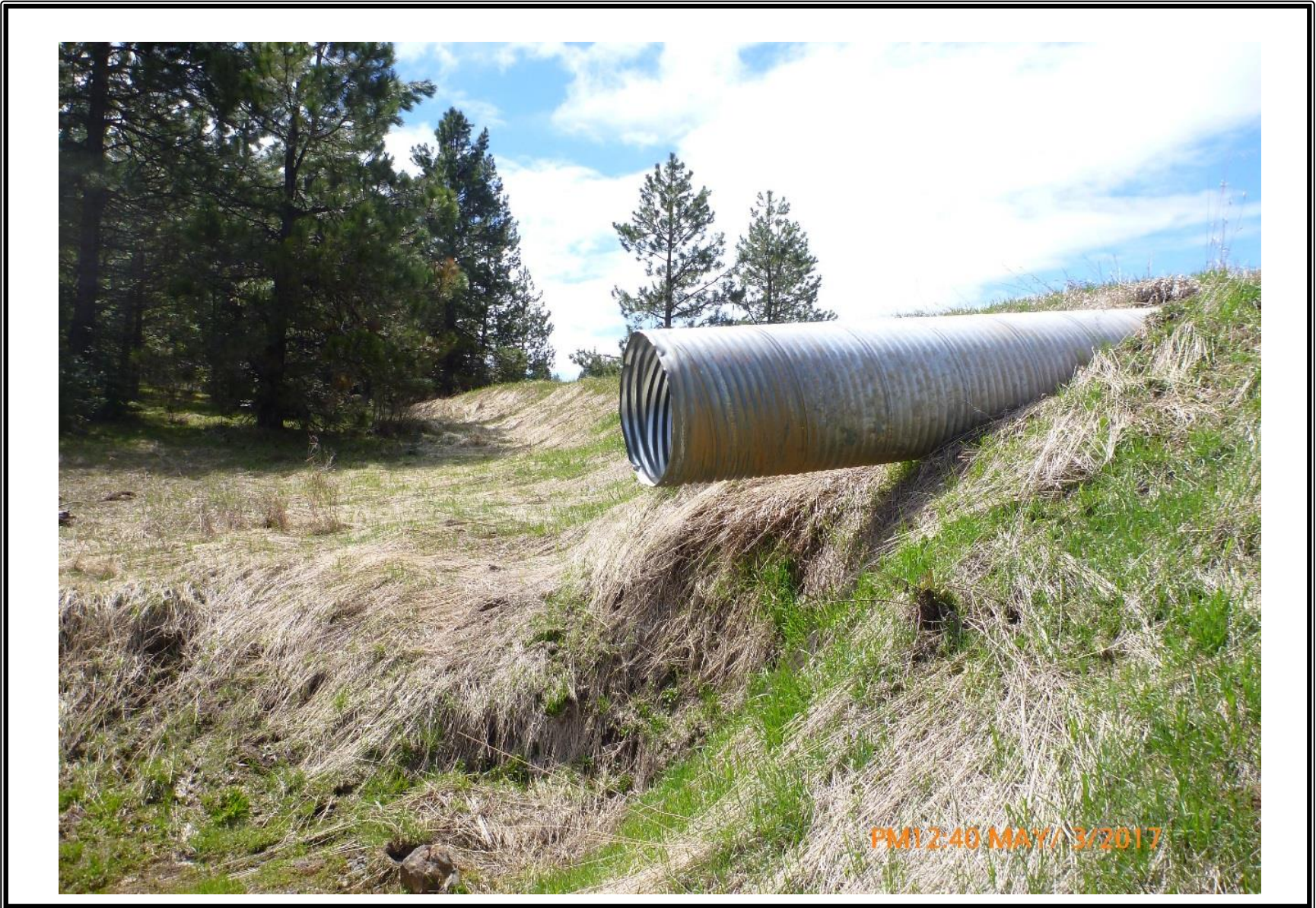
Figure 14. Downstream toe area at overflow spillway conduit. Notice erosion damage on slope
