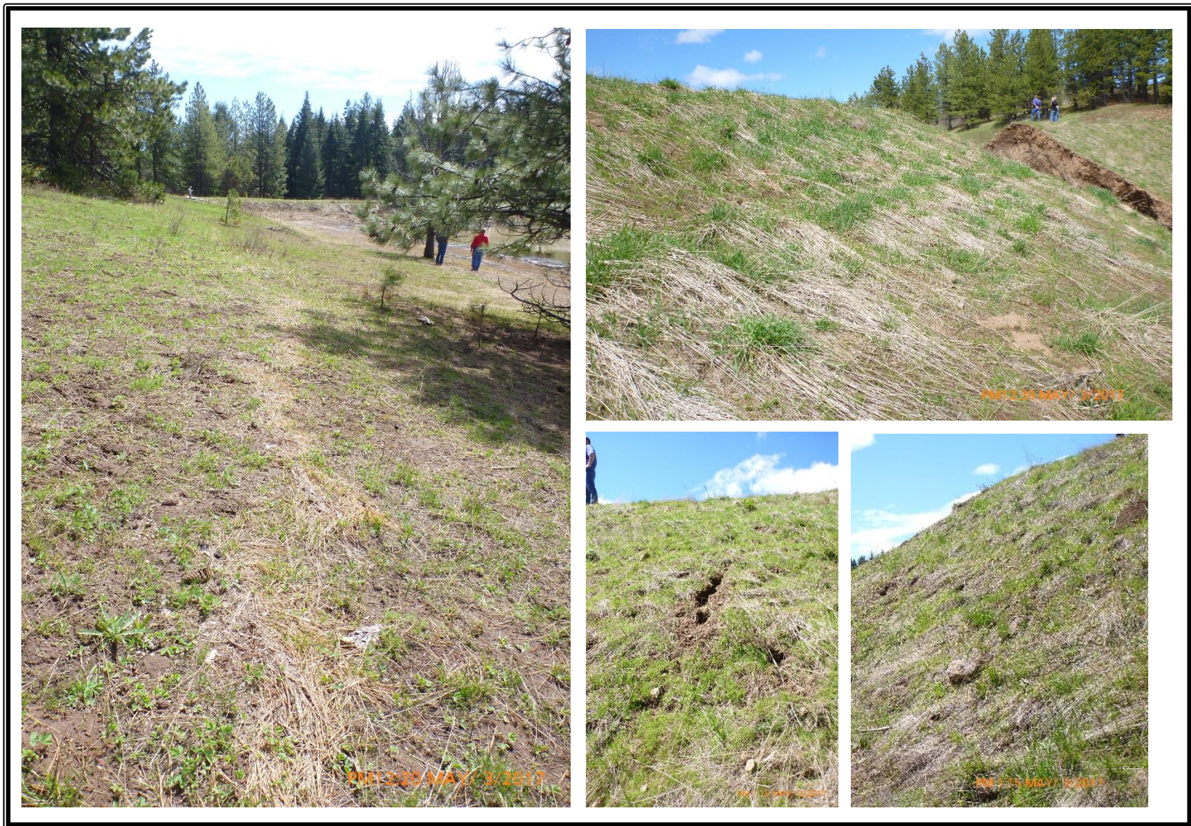
Figure 6. Bonasa Breaks Ranch Dam Inspection: debris line, grasses lying flat on the embankment, and erosion features.
