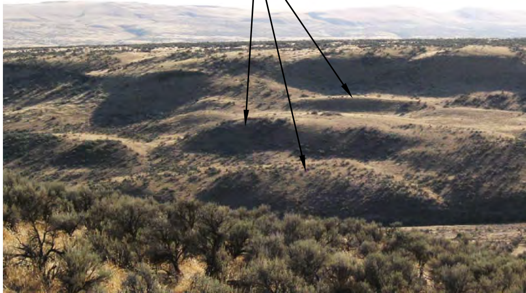
View to southeast at proposed right dam abutment area. Irregular benches and hummocky topography is a result of landslide failure of the Elephant Mountain Basalt unit over weak clay beds. Landslide deposits have covered the middle and lower slope units.
