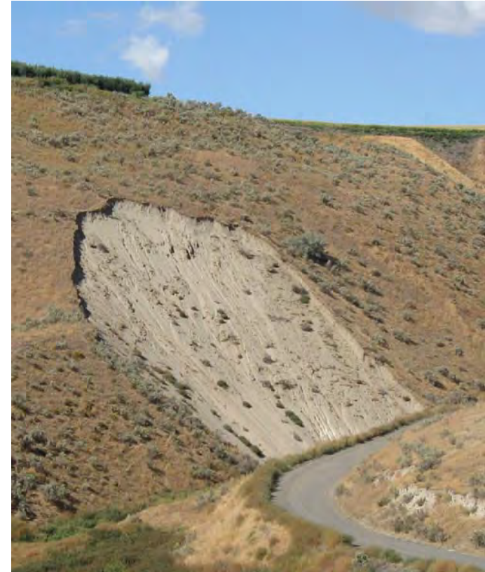
Shallow slope failure triggered by erosion at toe of slope. Similar failures may occur during reservoir filling and operation.
