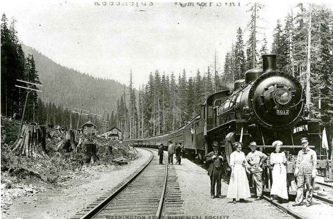
Figure 3-51. Keechelus Depot of the Milwaukee Road, ca. 1910
