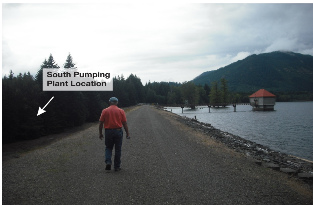
Figure 4-12. South Pumping Plant Location (South of Kachess Dam)
