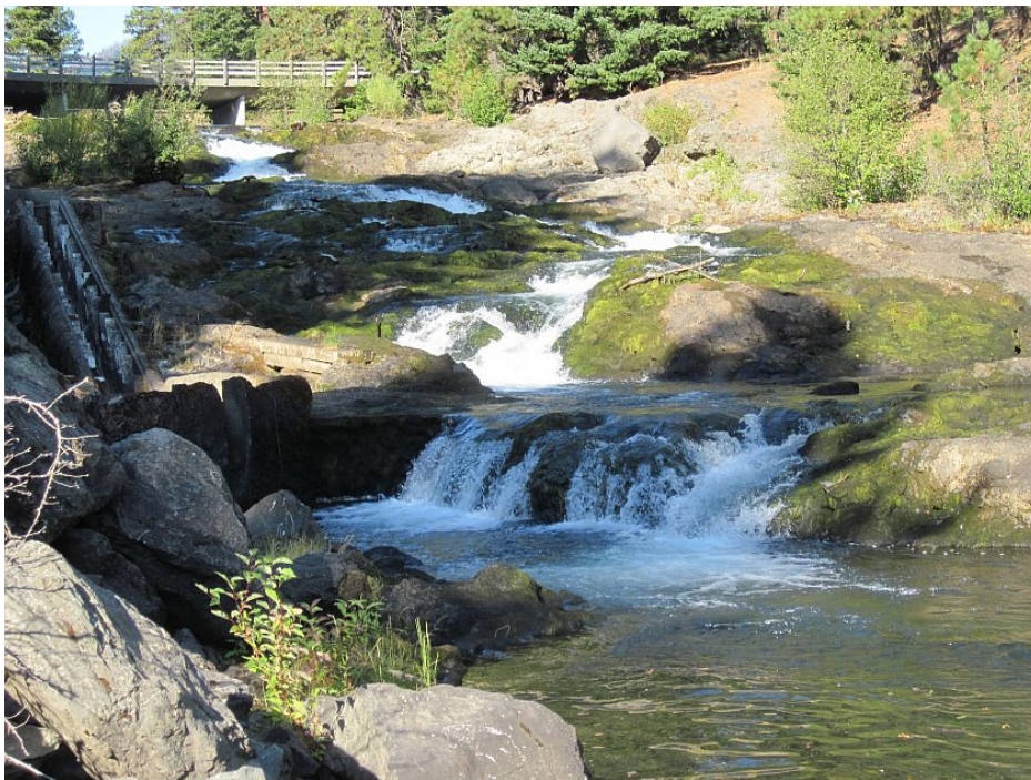
Figure 3-22. Clear Creek spillway on the downstream side of the spillway.
