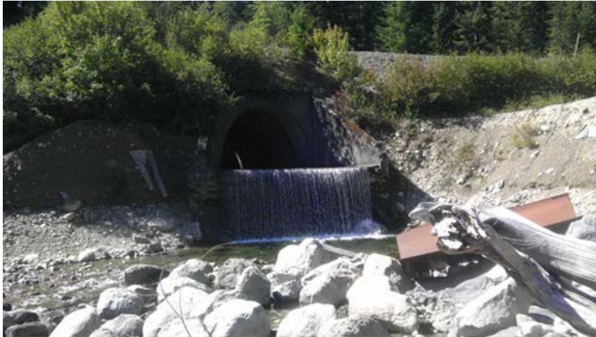
Figure 3-10. Existing passage barrier at Cold Creek culvert.
