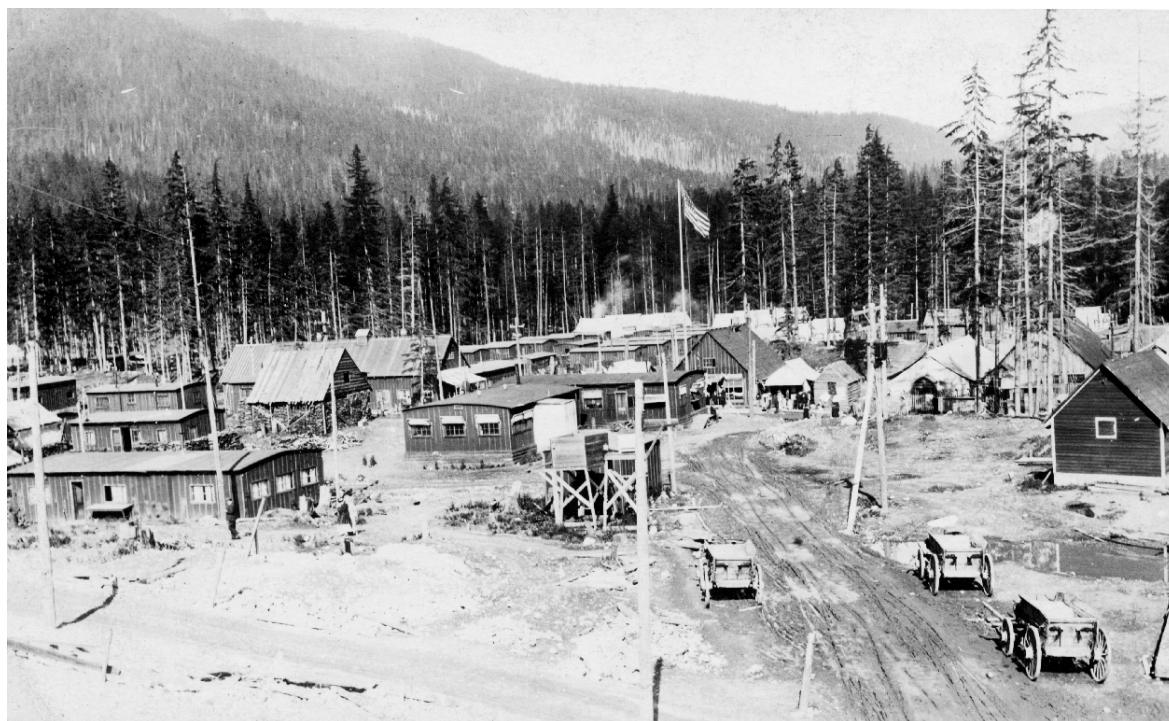
Figure 3-50. View of Keechelus Construction Camp ca. 1914.
