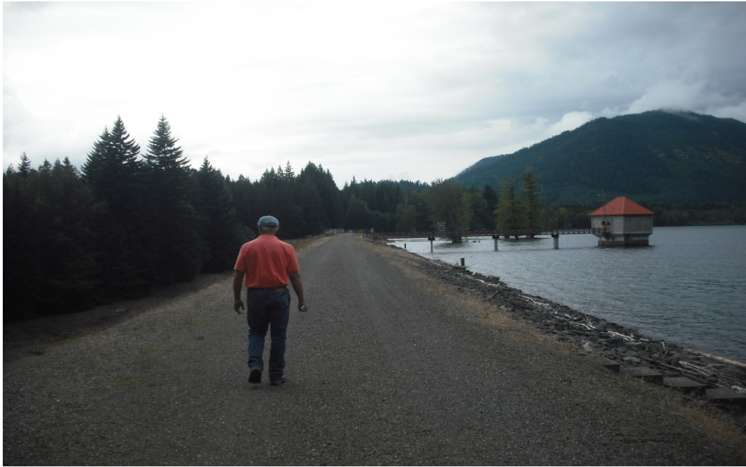
Figure 3-34. Kachess Dam – East End (at Dam) Facing West
