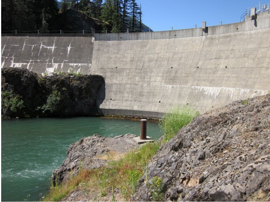
Figure 3-21. Clear Creek Dam on the downstream side of the dam.
