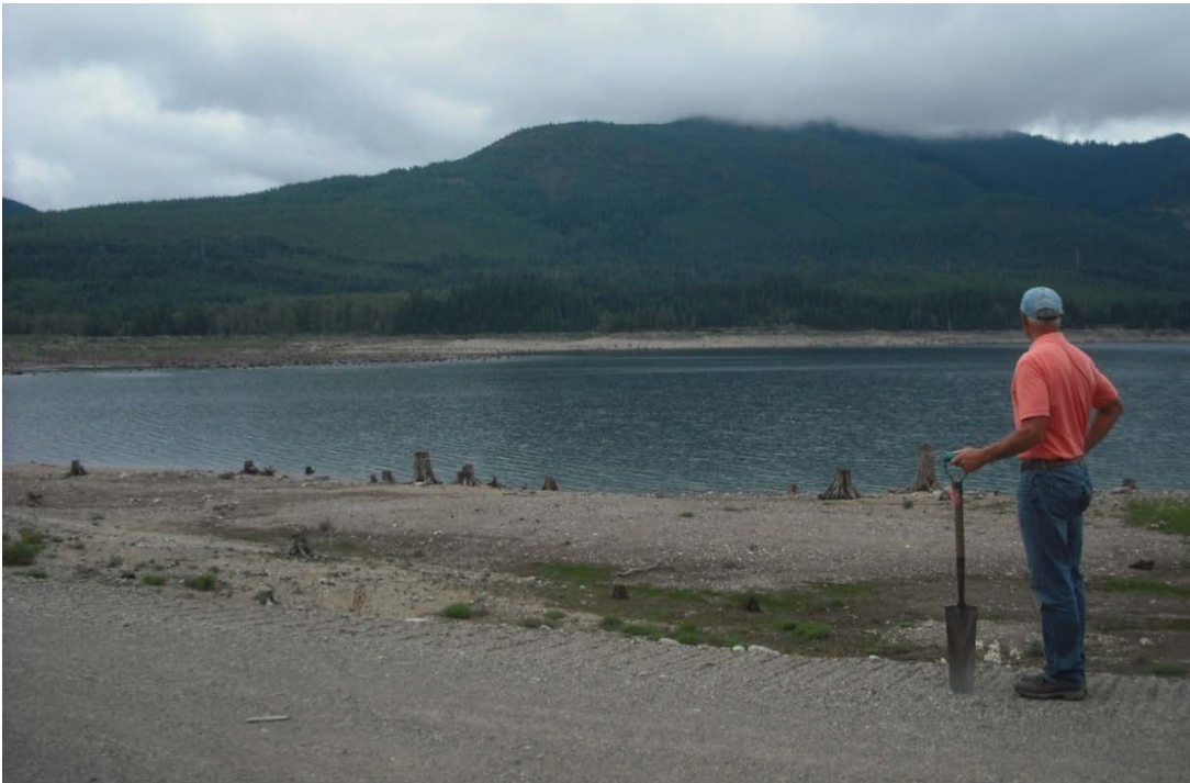
Figure 3-35. Keechelus Reservoir – South End (at Dam) Facing Northwest
