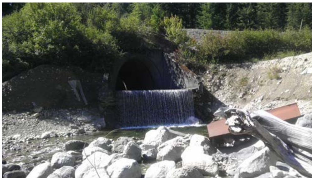
Figure 3-36. View of John Wayne Pioneer Trail and Cold Creek Culvert
