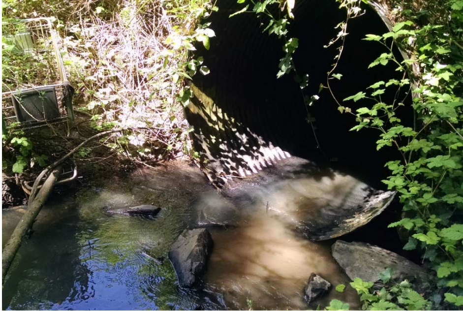
Figure 27. Looking downstream at site and culvert crossing under Hazel Dell Avenue.
