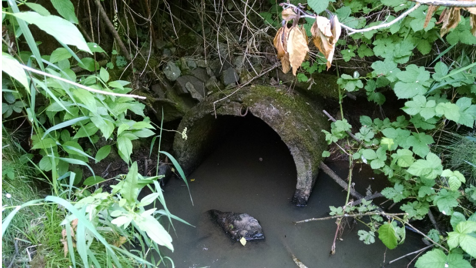
Figure 26. Looking downstream at WC_NE10NE149 site and culvert running under NE 10 th Street
