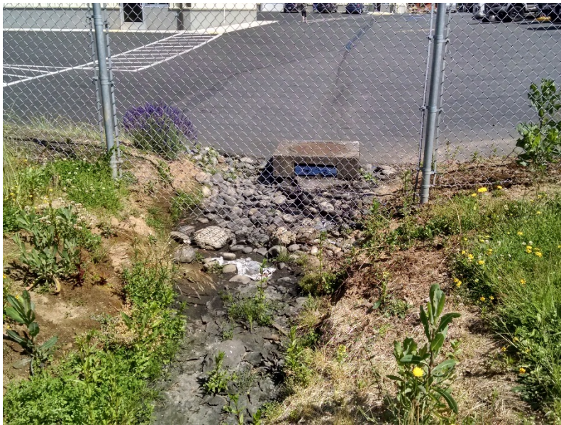
Figure 28. Detention basin inlet.
