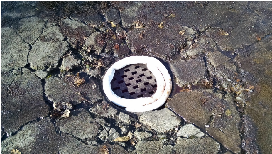
Figure 21. Dry weather reconnaissance of drain inlet, 9-7-2017.
