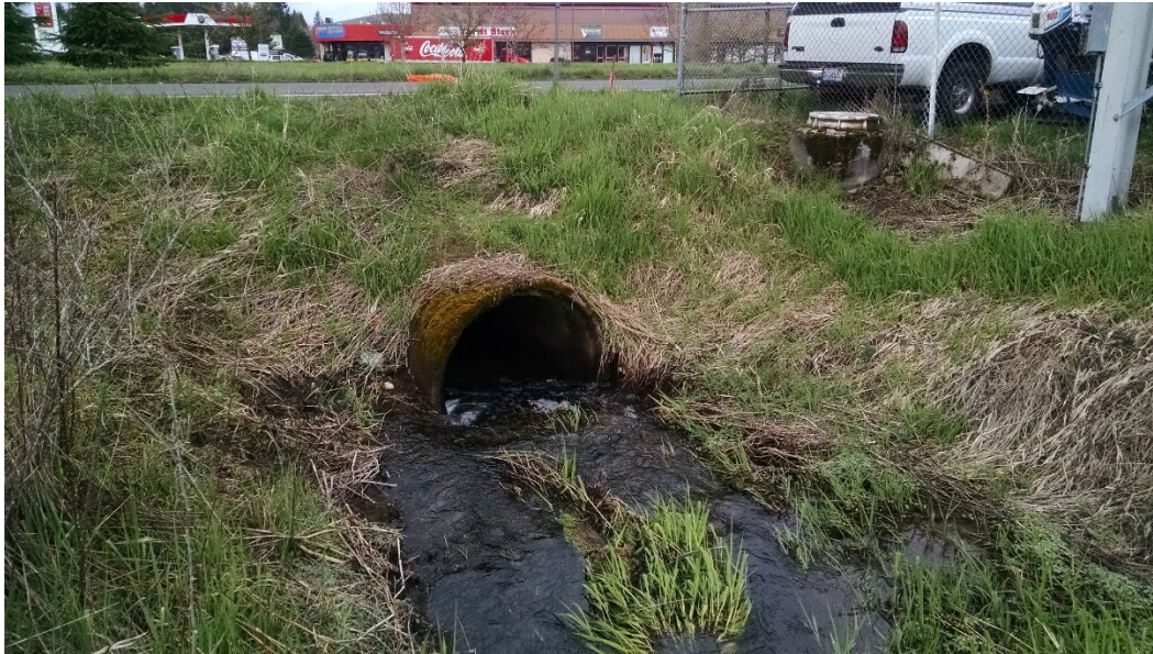
Figure 25. Looking downstream at St. Johns and Minnehaha Culvert site.
