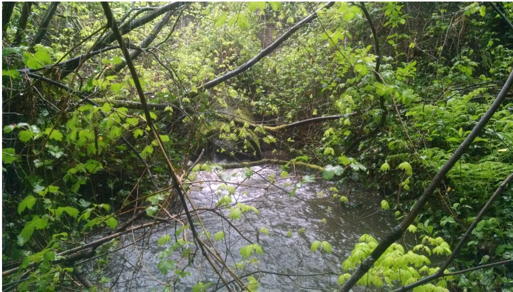
Figure 23. Looking upstream at culvert tributary, 4-24-2017.
